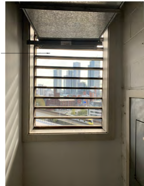
Existing hardwood timber slats with flyscreen mesh to 'open' vent area
