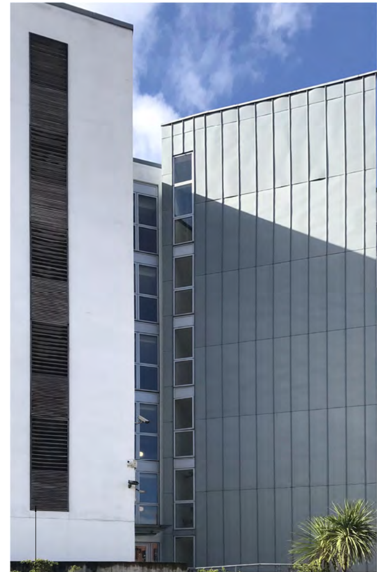
Existing louvre to refuse chute lobby.
