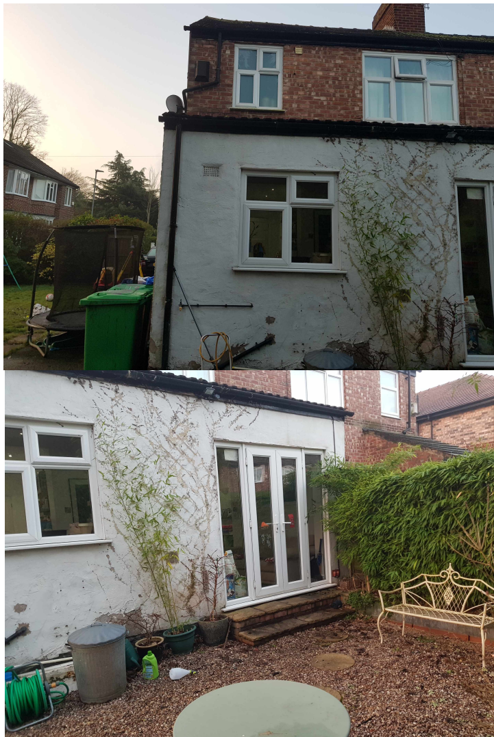
The existing lean to rendered extension adjacent to the courtyard.
