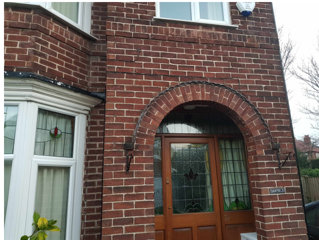
Original tile creasing over the arch and timber mouldings over bay window
