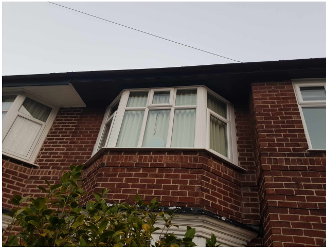
Brick detailing to the bay windows
