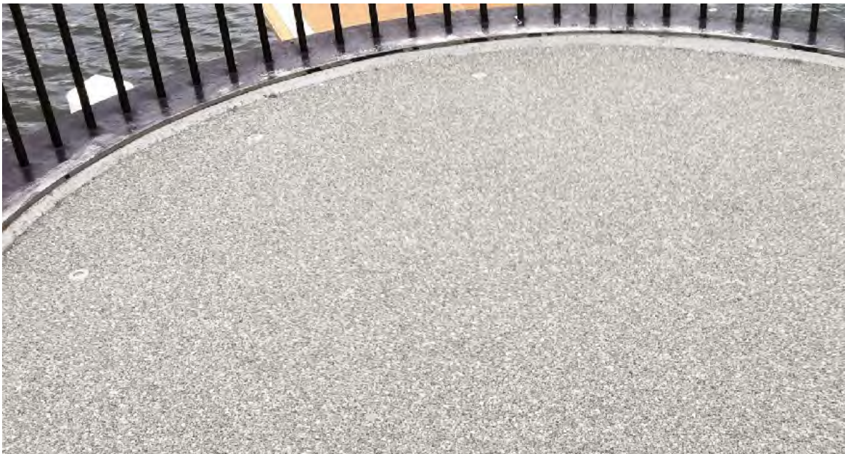
Example of a resin bound gravel bridge deck
