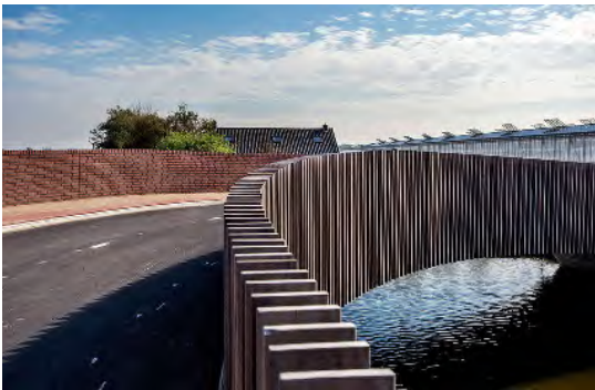
Individual regular timber elements Provide solidity and calming rhythm and minimise potential visual weight of balustrades by wrapping them into the deck
