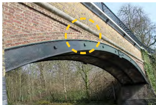
Exposed structure detailed to accentuate slender centre
