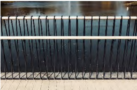
Simple repeating, elegant metal uprights with lower level leaning rail Ensures both pedestrians and cyclists feel considered and maximises views by utilising contrasting colours to help vertical element ‘disappear’ from the vista
