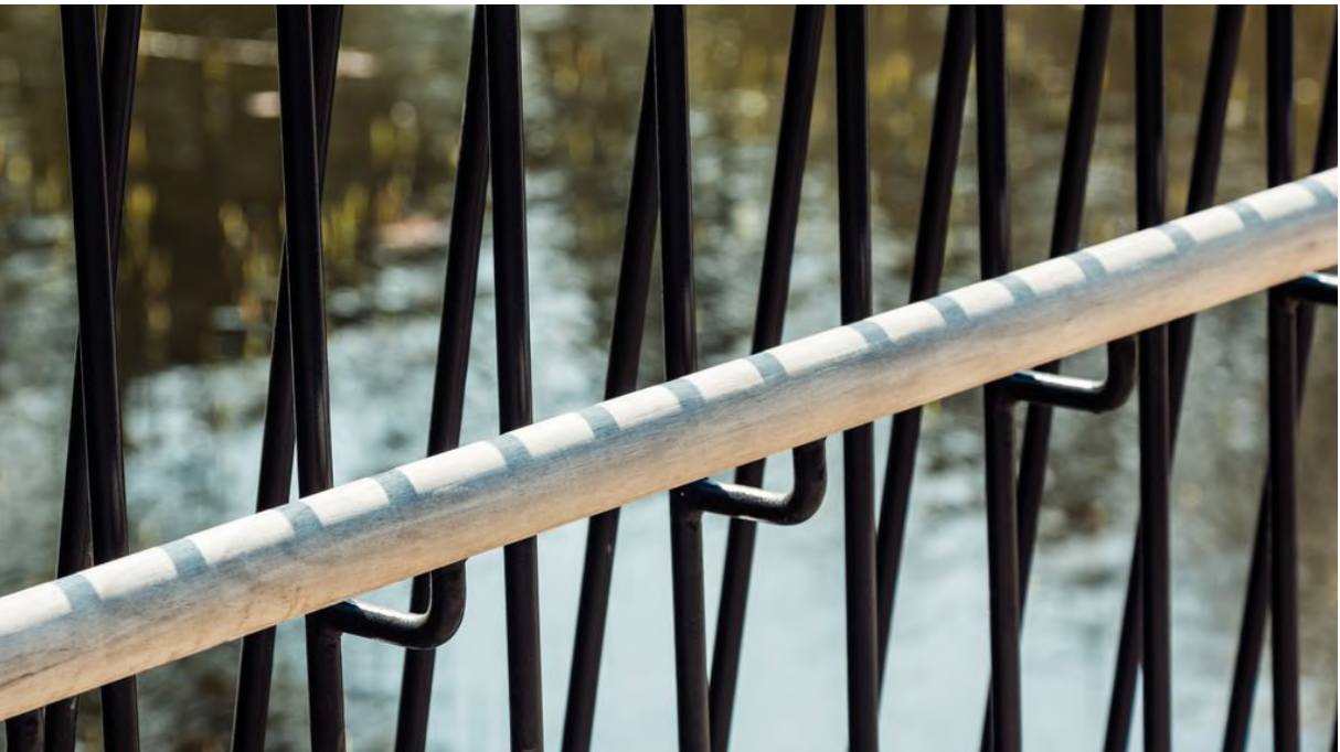
Woven Bridge, Copenhagen - Accoya handrail
