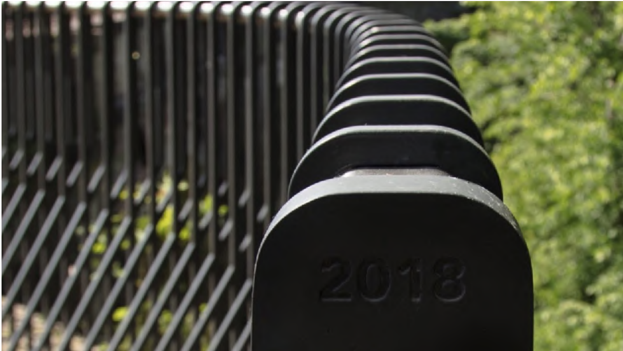
Marple Aqueduct - Powder coated steel balustrade
