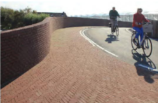
Paving Can be laid in different orientation to emphasise changes in direction and highlight movement flows
