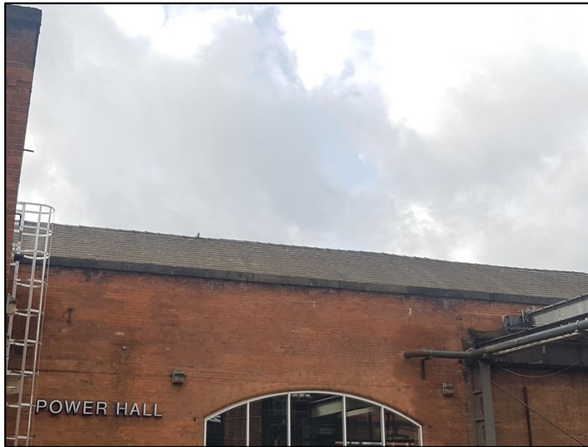
Photograph 4 showing the roof of the property
