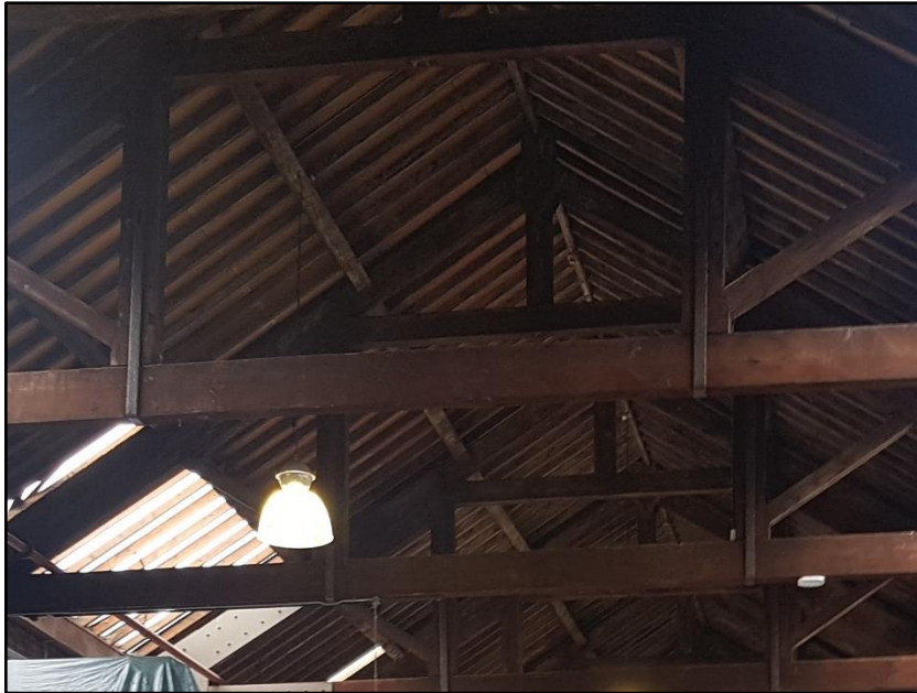
Photograph 8 showing the underside of the Power Hall roof
