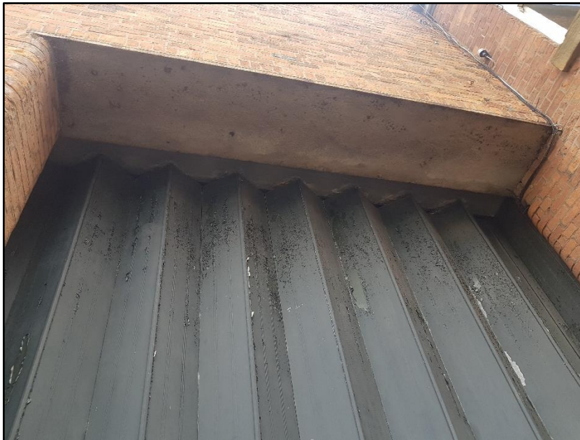
Photograph 3 showing the gaps above the folding metal cargo doors
