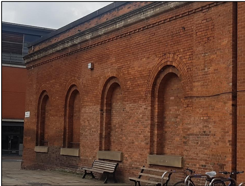
Photograph 1 showing the exterior of Power Hall
