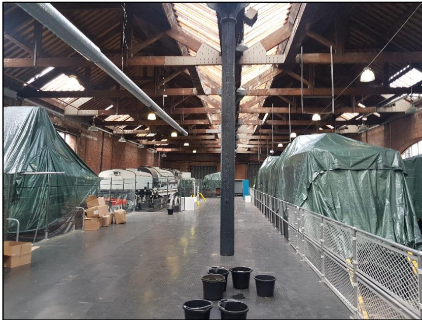
Photograph 6 showing the internal space open to the roof
