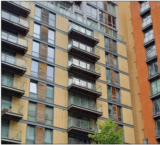
Existing Terracotta Tile
