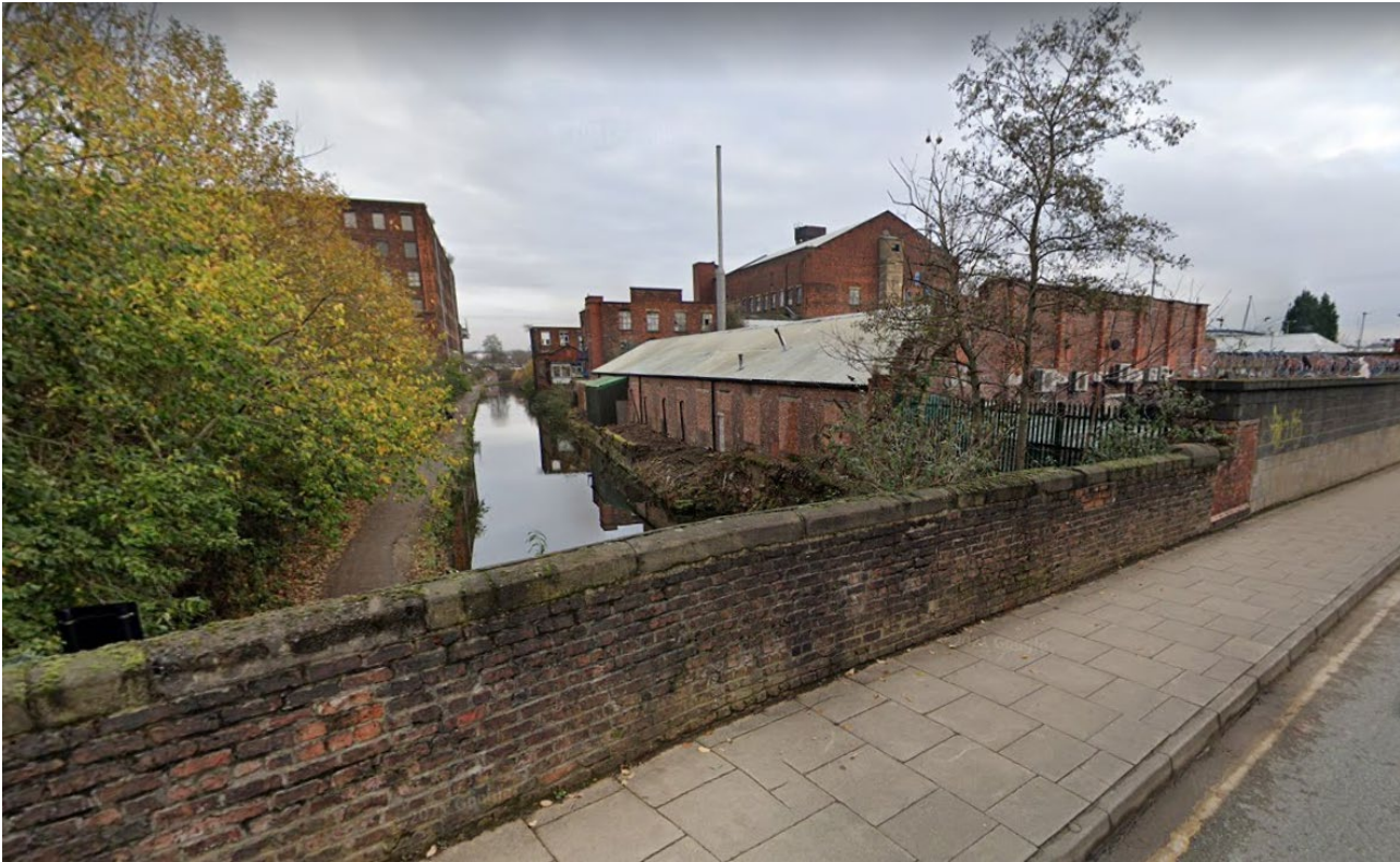
Rear View of PLT, showing canal, palisade fencing, and roofs.
