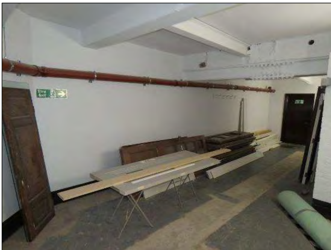
Figure 1d. The corner basement corridor space for the proposed offices.
