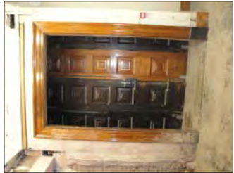
P5- Timber entrance doors
