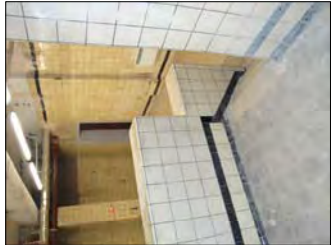
P4- Glazed tiling as seen throughout rooms B09, B10, B17, B18 & B19
