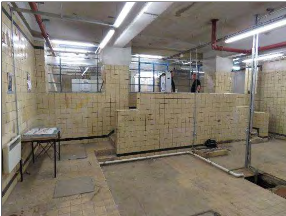
Figure 1c . The former Ventilating Plant room, with the main sump for all basement drains.
