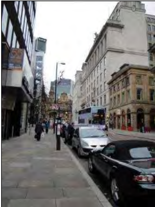
Figure 2: Long range view east along King Street illustrating: the scale, form and materiality of 100 King Street (right hand side) alongside that of the Ship Canal House
