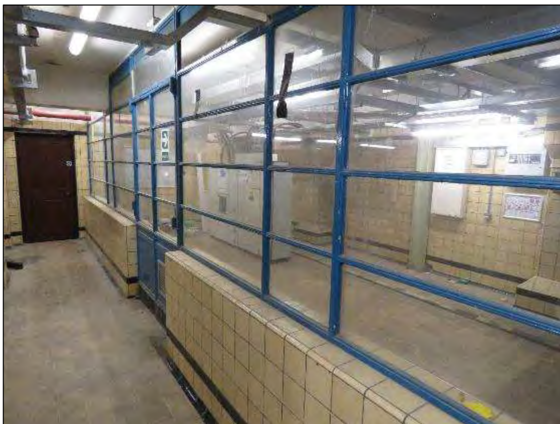
Figure 1b The glazed, metal-framed screen from the main plant room.
