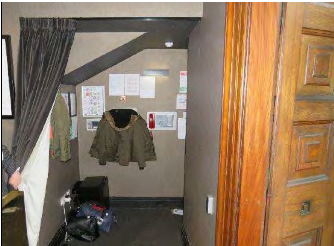
Figure 1i: The blocked former stair access to the basement, from the hotel entrance..
