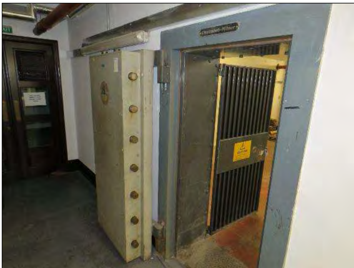
Fig 16a Strong Room doors – High significance - (June 2017) to be retained in situ.
