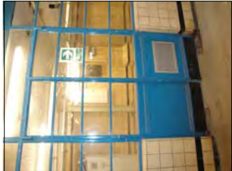
P2- Glazed wall and doors between rooms B09, B17 & B19
