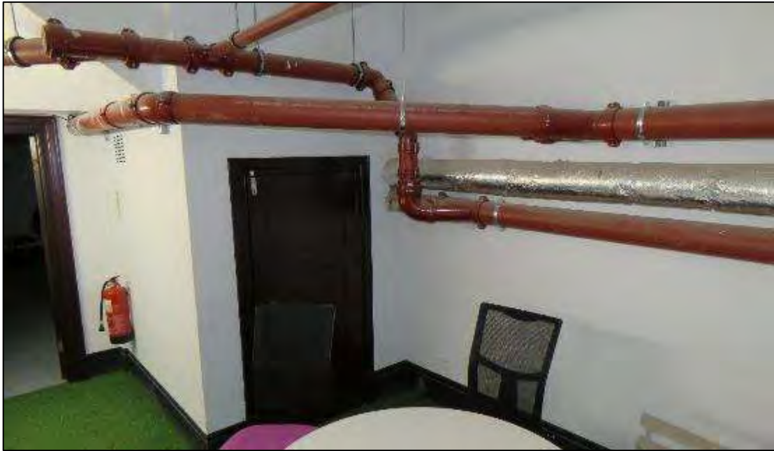
Figure 1h. Corner of the corridor, currently used as staff meeting space.
