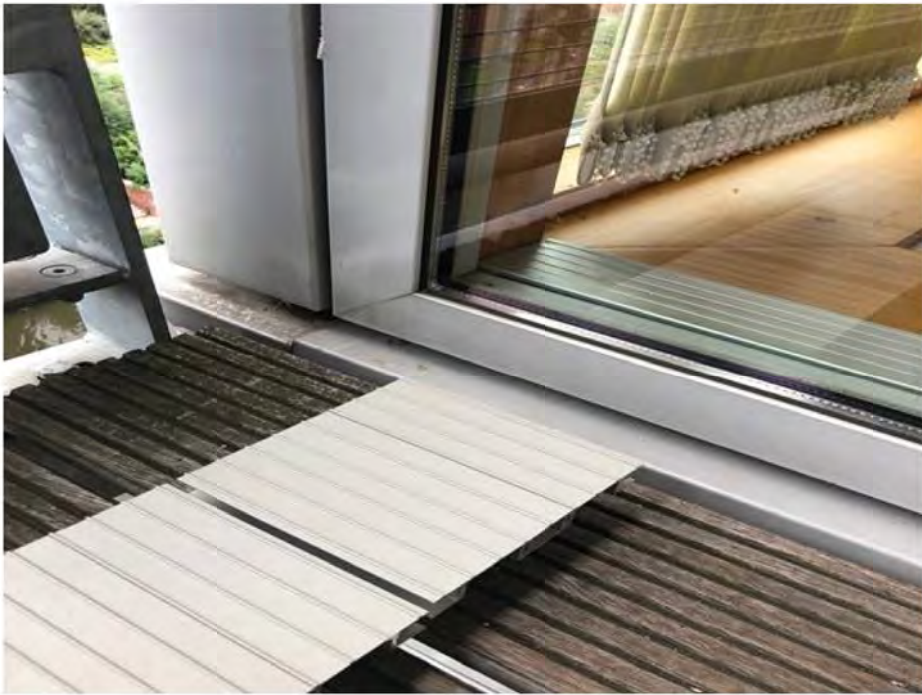
Existing decking with AliDeck sample. Please note this is RAL 7030 Stone Grey. not the proposed RAL 7039 Quartz grey
