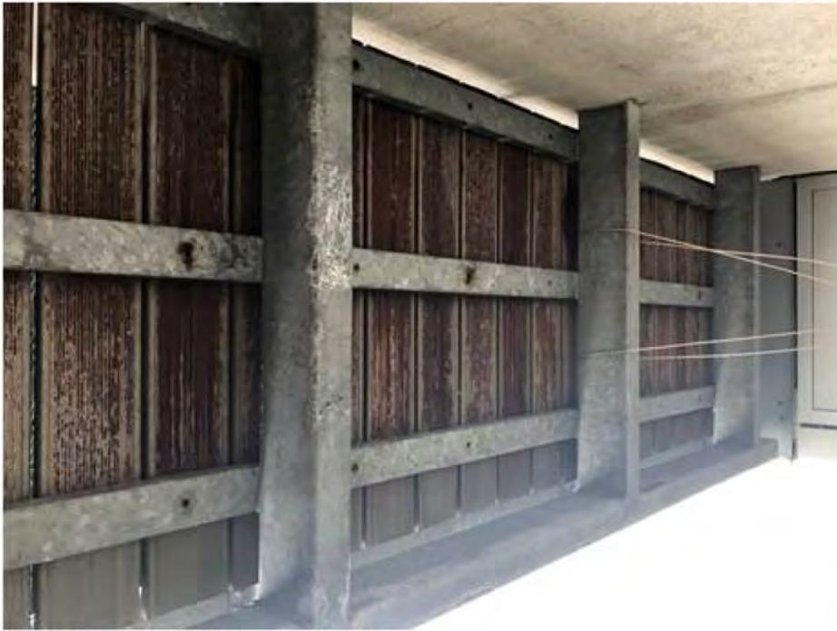
Existing decking underside
