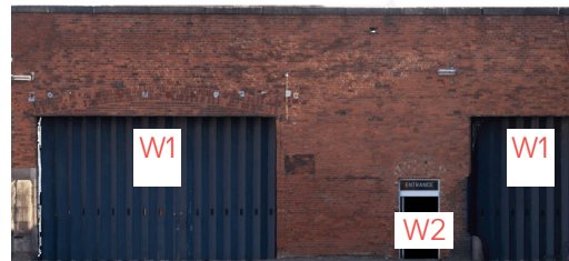
Upper Yard West 1
