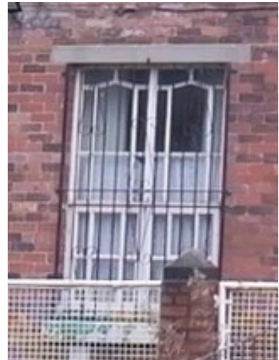
Existing window at front elevation
