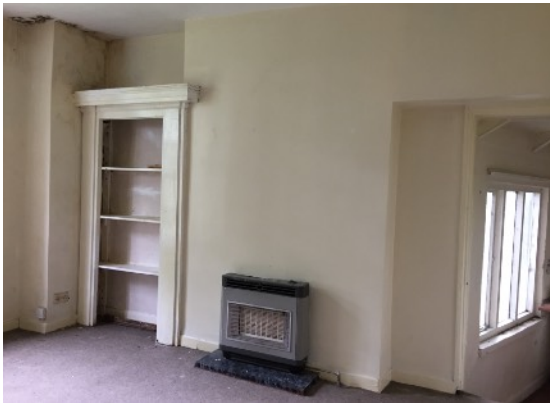
Existing chimney breast with electric heater
