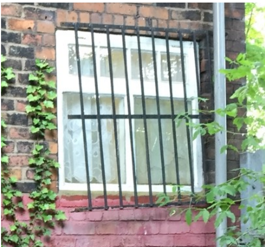
Existing window at side elevation
