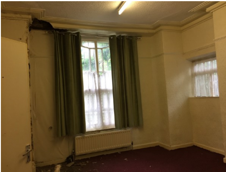
Room 1 looking towards front elevation
