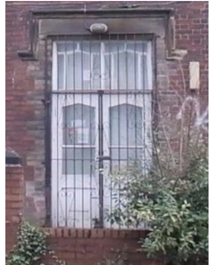
Access doors at front elevation
