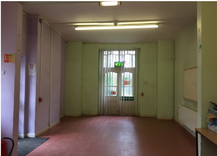
View towards front access doors
