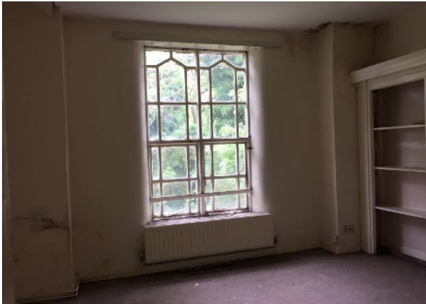
Room 5 looking towards front elevation
