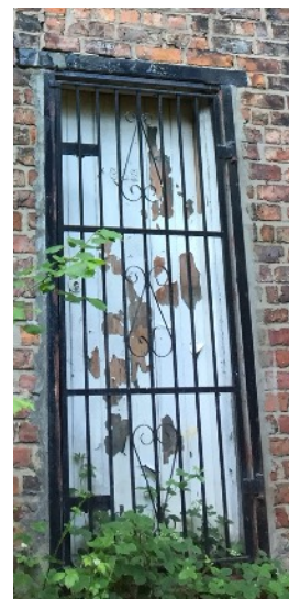
Exit door to side
