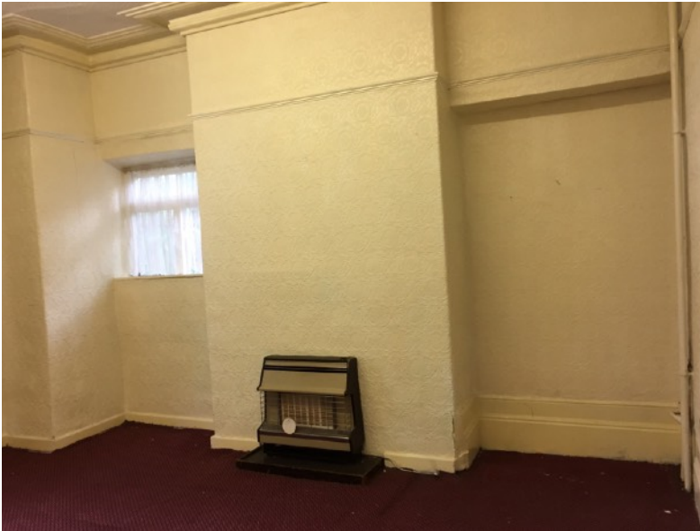
Existing chimney breast with electric heater
