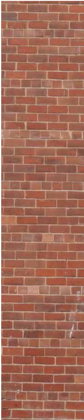
Existing Brick Facade
