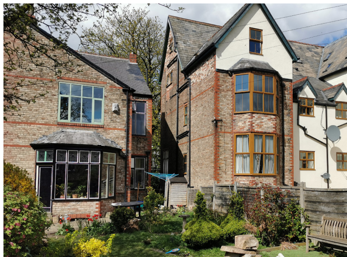
As existing from the rear
