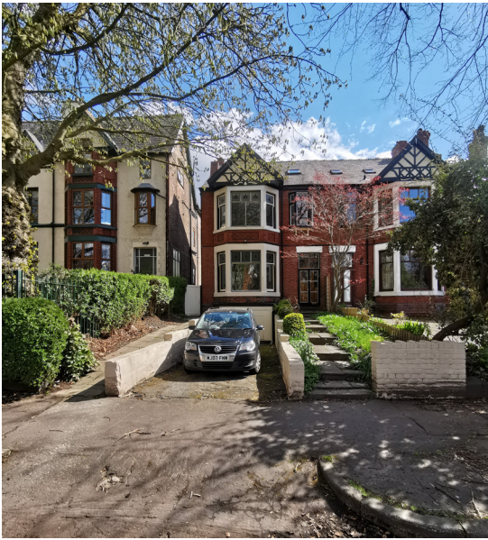
15 Whalley Road viewed from the front
