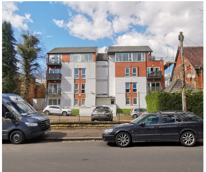
Block of flats directly opposite 15 Whalley Road
