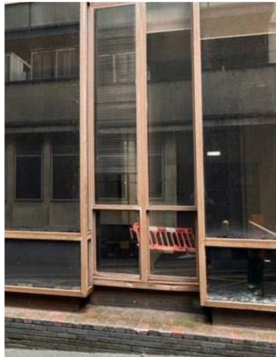
Figure 27a: The condition of the original windows to the Marsden Street elevation in 2022.
