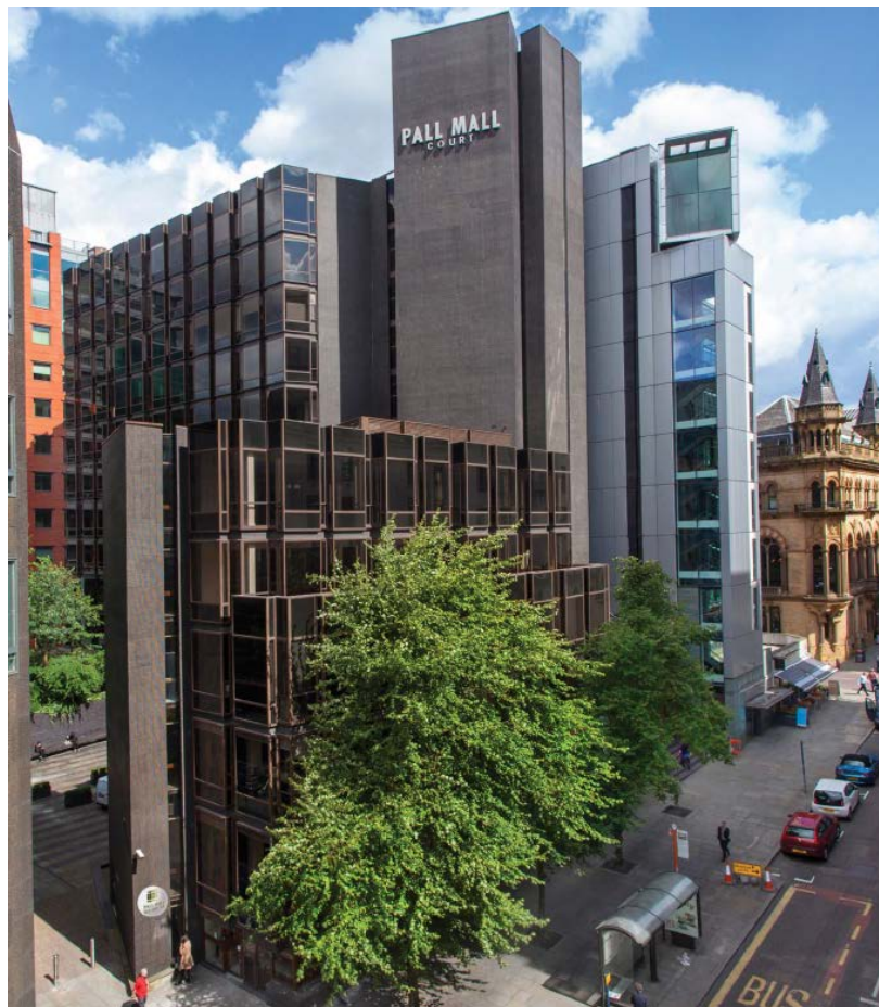
Figure 1: Pall Mall Court looking east along King Street.
