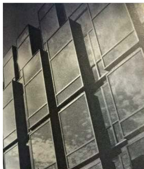
Figure 26: 1970 - A typical section of glazed bays. Note the paired bays separated by single and pairs of recessed, metal frame sash windows.
