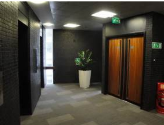
Figure 38: An example of a lift lobby, showing the original mosaic walls with black cement pointing and double doors into the King Street Block. The carpets were installed in c2003, along with the suspended ceiling and lights. (Photo taken in 2017; condition has since deteriorated)
