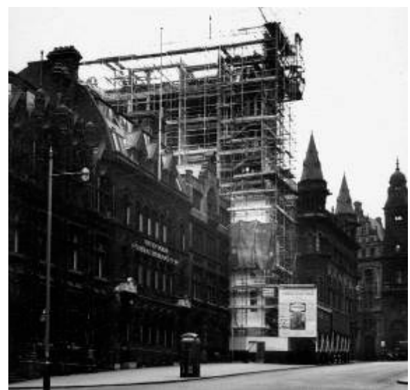
Figure 21: Jan 1960 – The new Norwich Union Offices (adjoining Pall Mall Court) in the process of construction.
