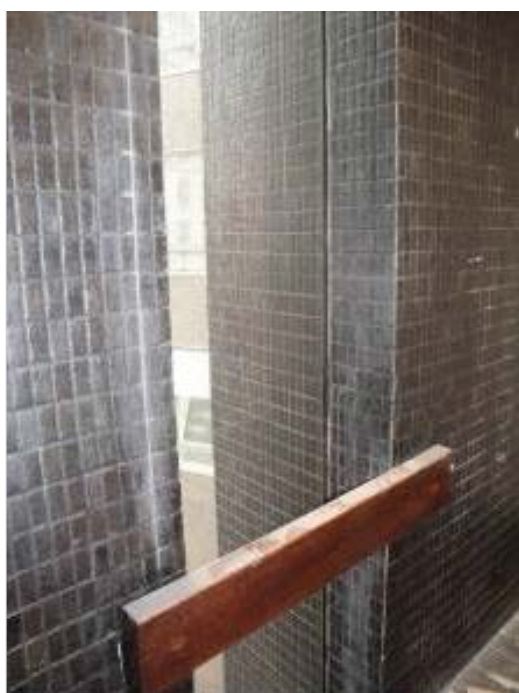
Figure 34: An example of the attention to detail in the lift lobbies on each floor, a single piece of bronzed glass is inserted directly into the window jambs creating the illusion of the internal and external tiled surfaces being uninterrupted. (Photo taken in 2017; condition has since deteriorated)
