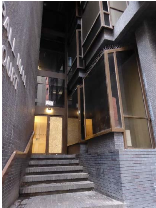
Figure 27: The condition of the Marsden Street Entrance in 2022.
