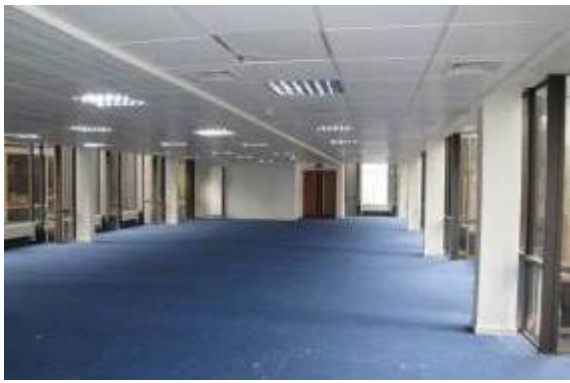
Figure 45: A typical king Street Block office floor showing the modern carpet, modern lowered suspended ceilings and lighting. (Photo taken in 2017; condition has since deteriorated)
