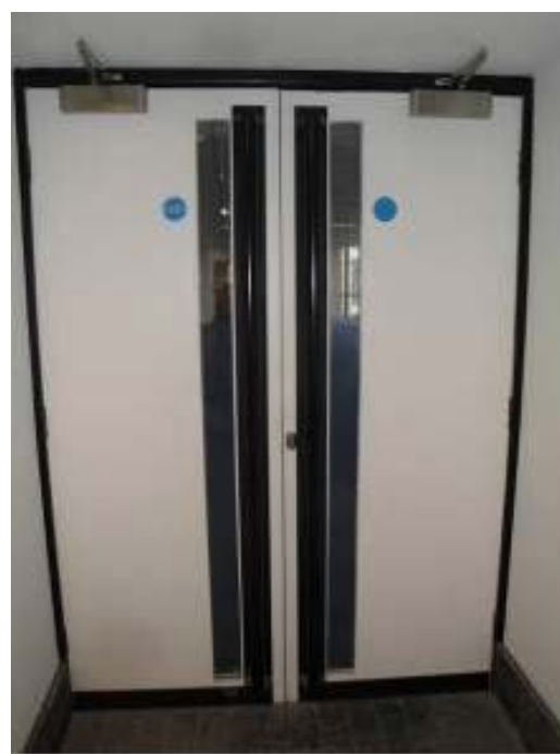
Figure 35: An example of a typical pair of original melamine covered internal doors, separating the main office space from the fire escape core. (Photo taken in 2017; condition has since deteriorated)
