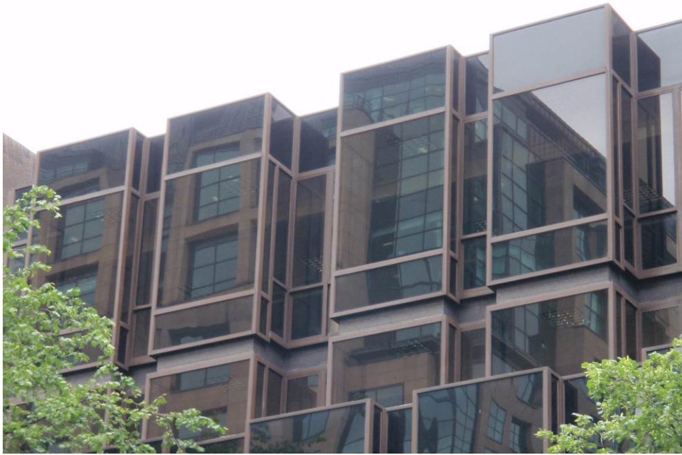
Figure 27e: An example of the original windows to the upper parts of the building facing onto the piazza, which comprise an undulating system of oriel windows. Note the use of narrower single-glazed spandrel panels and the continuation of small black mosaic tiles used between each floor level (Photo taken as seen in 2017; condition has since deteriorated)
