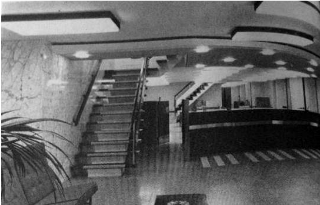
Figure 40: The entrance of the Bank of America, entered from Marsden Street.c1970
