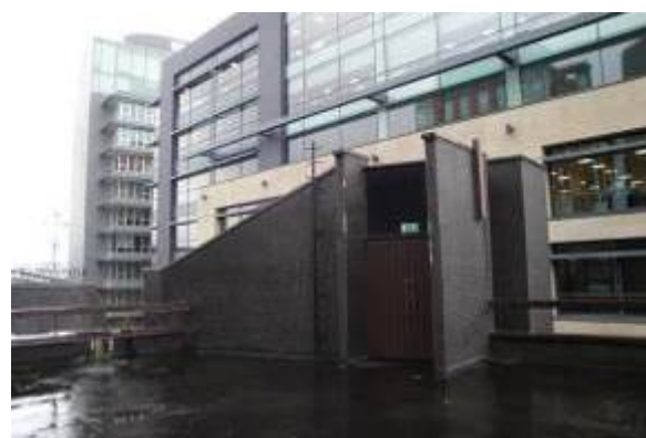
Figure 51: The eastern fire escape core which acted as the fire escape for the caretakers flat. (Photo taken in 2017; condition has since deteriorated)
