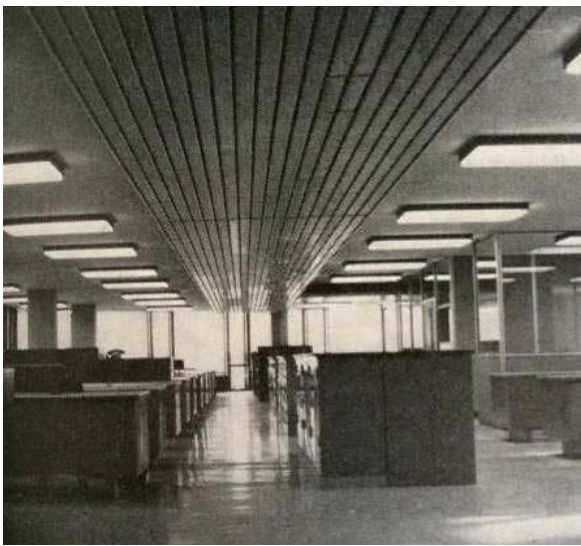
Figure 42: A typical floor layout looking north in the Central Block. Note the beige vinyl floor covering and original metal boards denoting the central ‘corridor’. C1970
