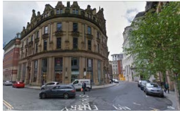
Figure 61: A view looking south along Spring Gardens, to the right, and York Street to the left.
