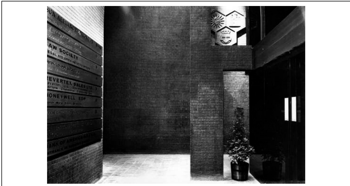
Figure 46: The entrance foyer, looking east in 1969, note the original glazed doors to the right and extent of mosaic tiles and Staffordshire blue engineering brick. To the top right of the image is the Sun Alliance sculpture by Josephine Reid.
