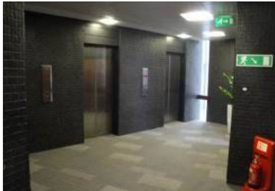
Figure 36: An example of a lift lobby connecting the Central Block to the King Street Block, showing the survival of the original mosaic walls with black cement pointing. The carpets were installed in c2003, along with the ceiling and lights. (Photo taken in 2017; condition has since deteriorated)
