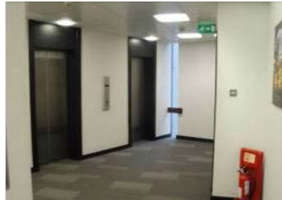
Figure 37: An example of a lift lobby connecting the Central Block to the King Street Block, showing the replacement of the original mosaic tiles with plastered surfaces. (Photo taken in 2017; condition has since deteriorated)
