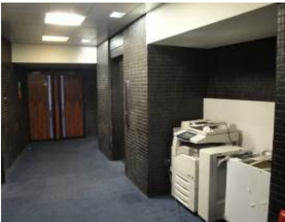
Figure 39: An example of a lift lobby which connects the Marsden Street Block to the Central Block, showing original tiling, black cement pointing and doors. (Photo taken in 2017; condition has since deteriorated)
