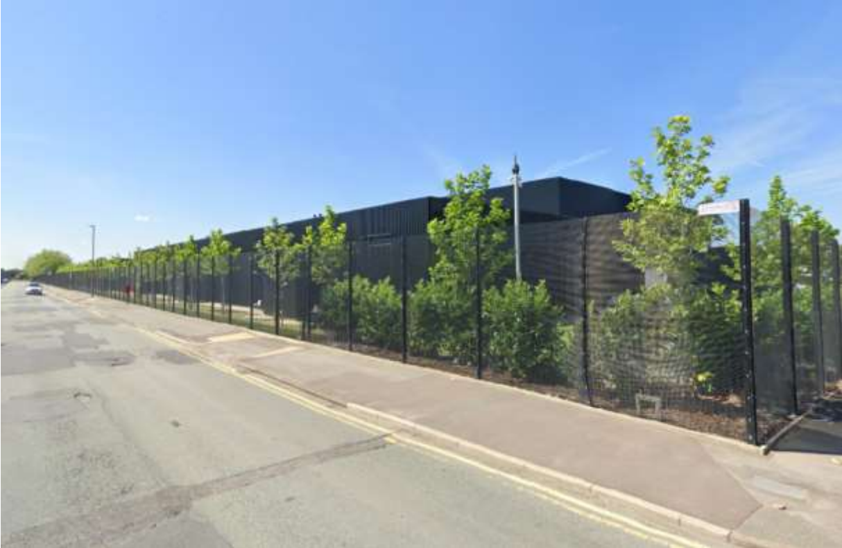
Outer Space Studios from Wenlock Way looking west
