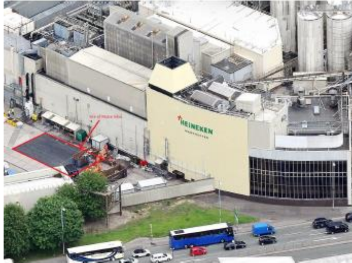
Aerial view looking east towards application site edged red
