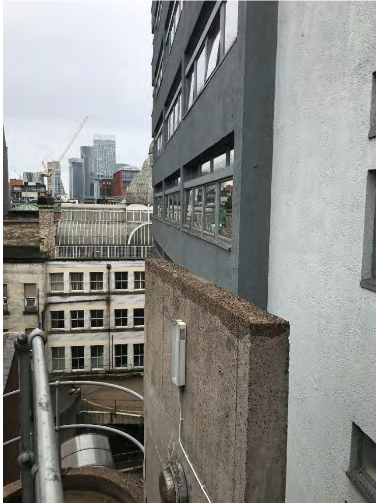
Photo 4: Overlooking onto adjacent plot Barton Arcade
