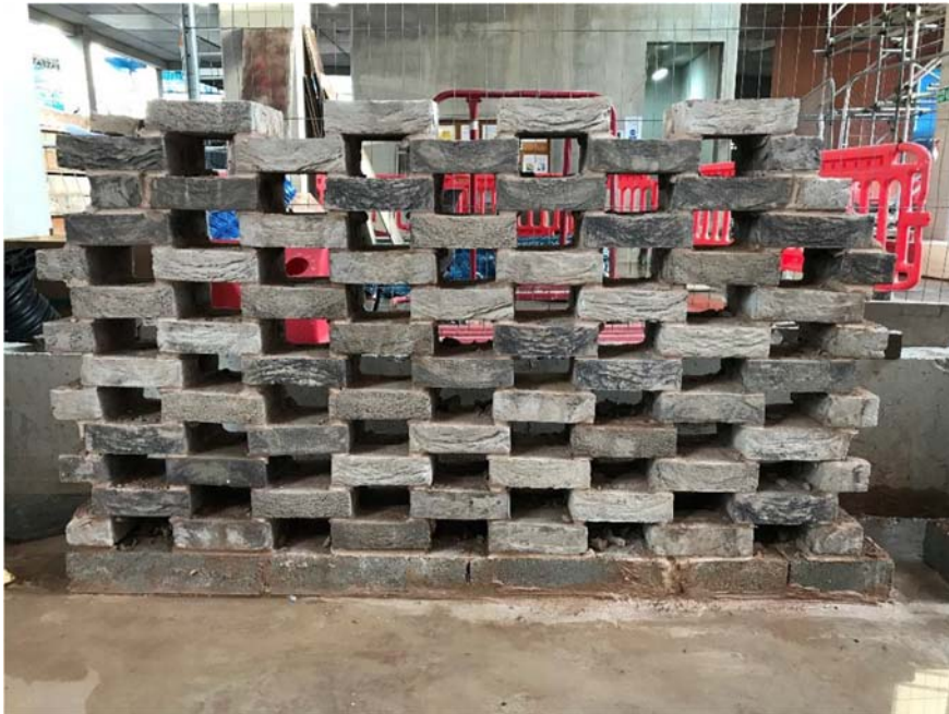
Hit and Miss Brickwork
