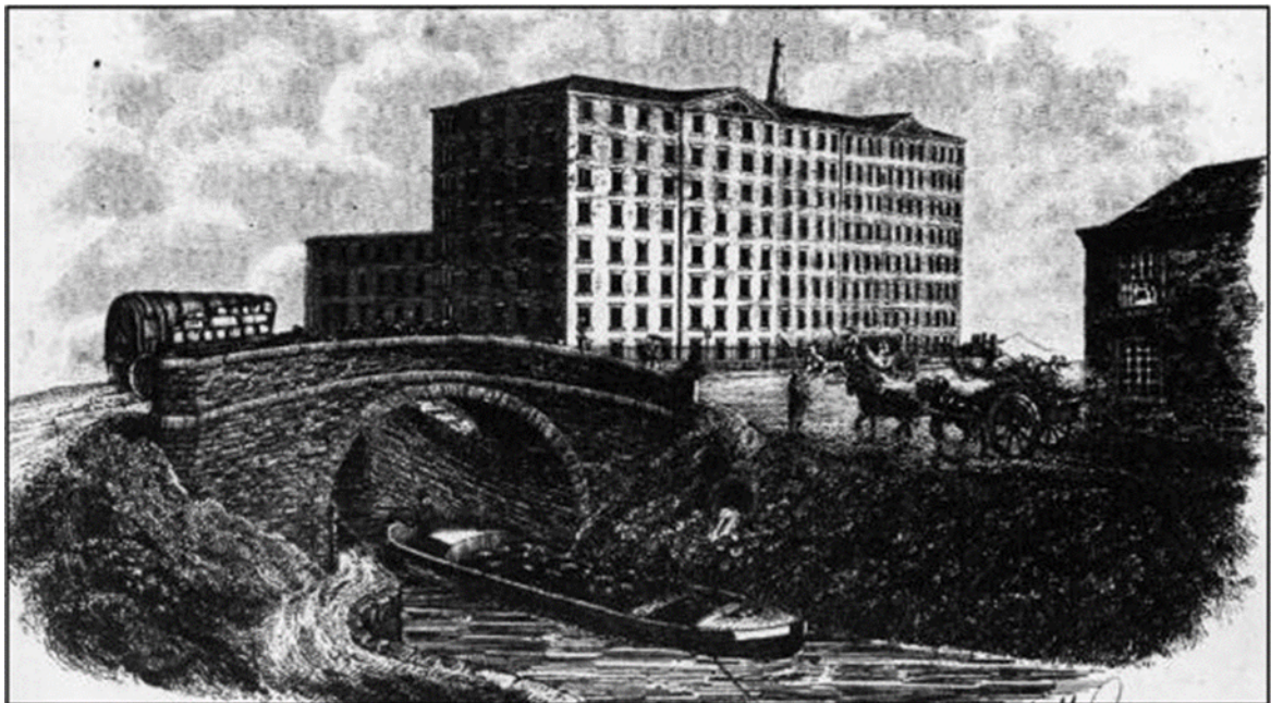
Figure 10 Pollard Street Mill, Great Ancoats Street, 1825, with Ashton Canal in foreground. The bridge in the foreground is likely to be the same location as the current bridge at Lock 1, carrying what is now Great Ancoats Street; however, both bridge and road have changed significantly since that time.
