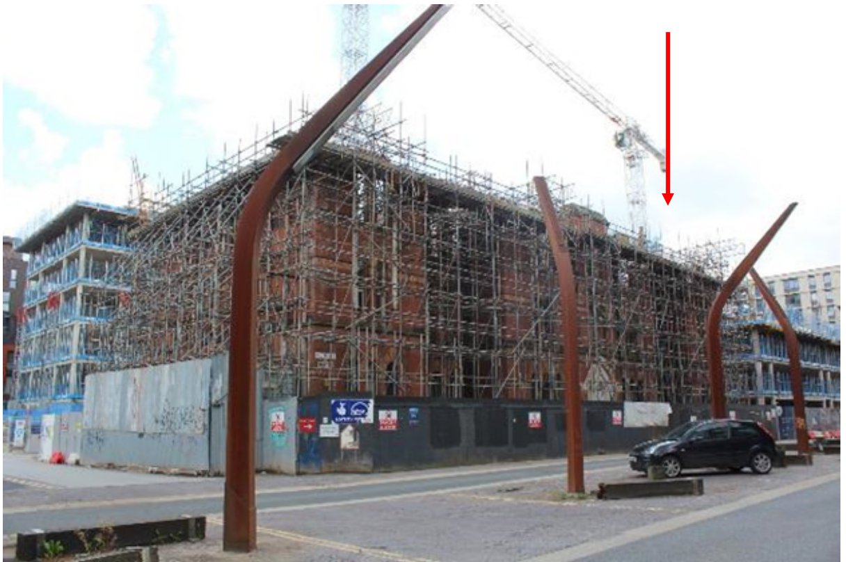
Figure 26: Asset no. 11 – Ardwick and Ancoats Hospital, on Old Mill Street looking south towards the Site (indicated by red arrow) (Authors Own, 2020)
