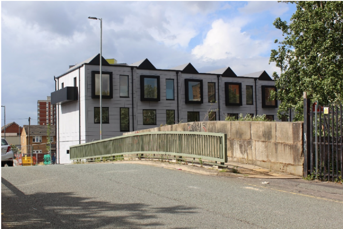
Figure 27. Asset no. 8 - Bridge Number 5 Over Ashton Canal looking North West away from the Site (Authors Own, 2020)
