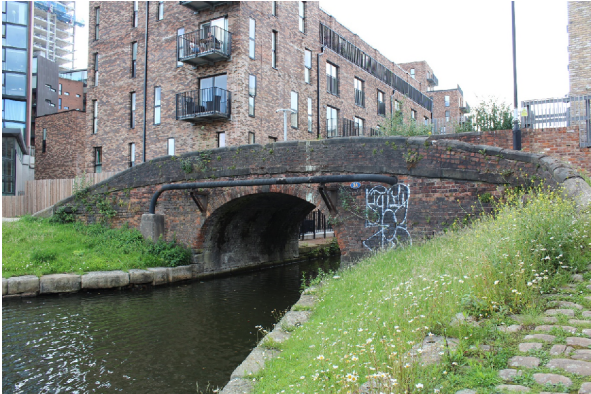
Figure 32 Canal Towpath Bridge (Authors Own, 2020)
