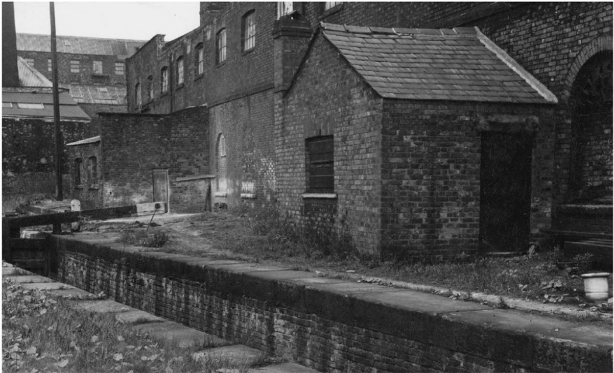
Figure 17. Soho Foundry Wall, 1960, with Lock 2 in foreground (Manchester City Council Libraries) As can be seen, much of the structure here can still be viewed today, and is one of the few remaining elements of the industrial buildings which previously defined the context of the canal. However, the buildings in the background, likely the remaining elements of Soho Foundry, have since been demolished.
