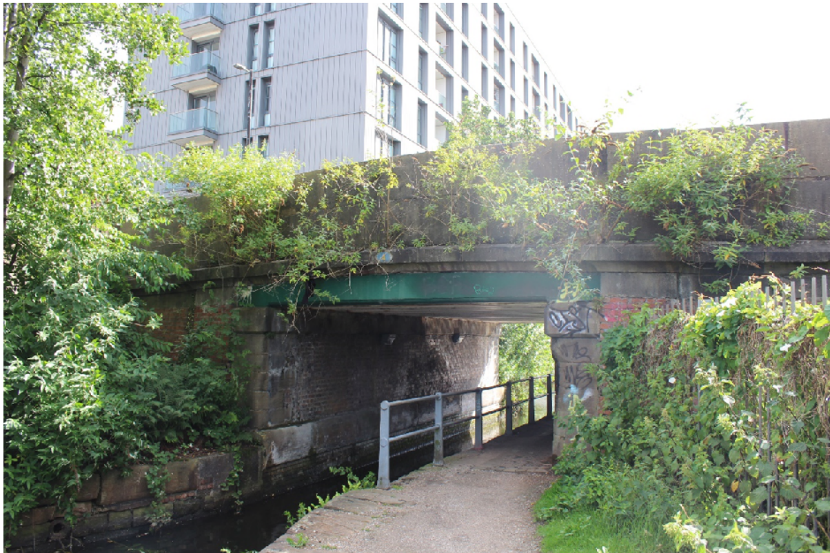
Figure 38: Bridge Number 4 Over Ashton Canal (Authors Own, 2020)
