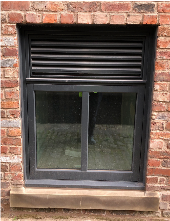
fig01: example of louvre to head of window arrangement to canal street elevation of minto & turner. sample as viewed on site.
