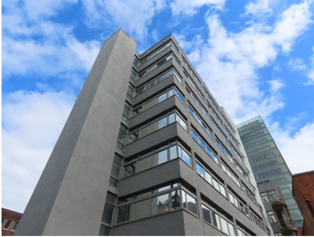
Photograph 1 - Building facade showing concrete construction with relatively recent cladding.
