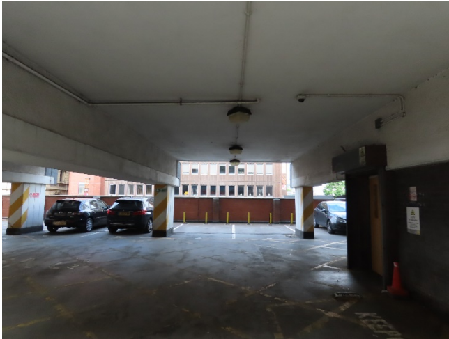
Photograph 3 - Semi-open car park comprising 3rd Storey.
