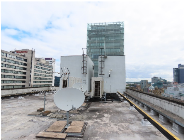
Photograph 2 - Example of flat rooftop atop 39 Deansgate.
