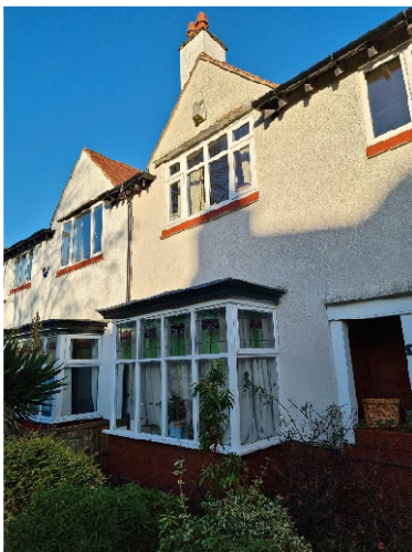
Fig 1 – View of front of property
