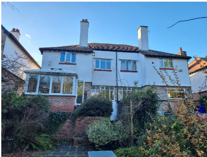
Fig 2 – View of rear of property
