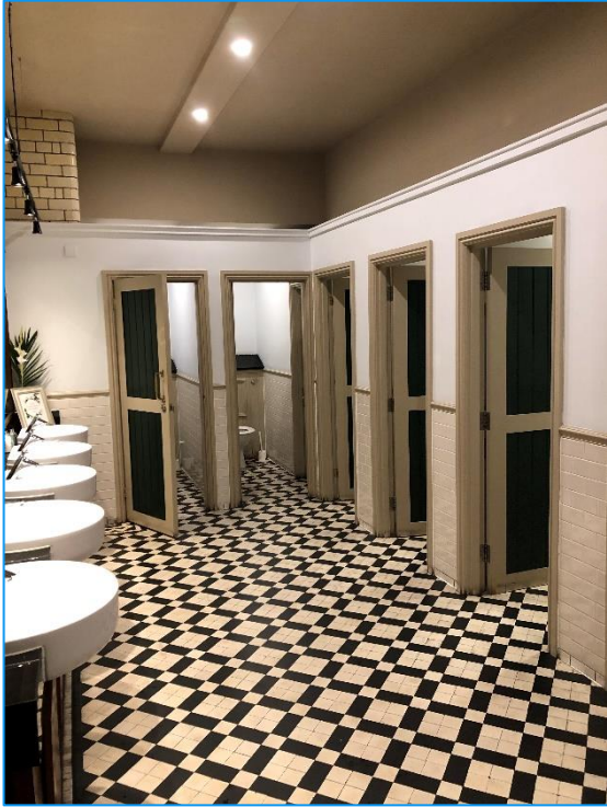
Figure 21: Ladies Toilet created a decade ago.
