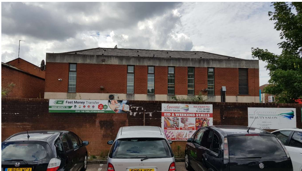
East (rear) elevation of the application site showing the harsh slab sided nature of the original architecture
