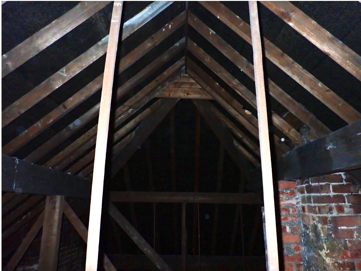
3.2a – The roof void.
