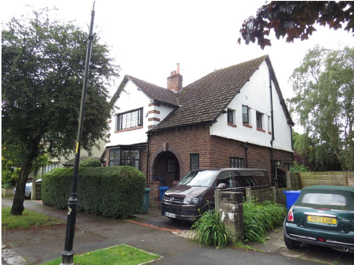
3.1a – The front of the house.
