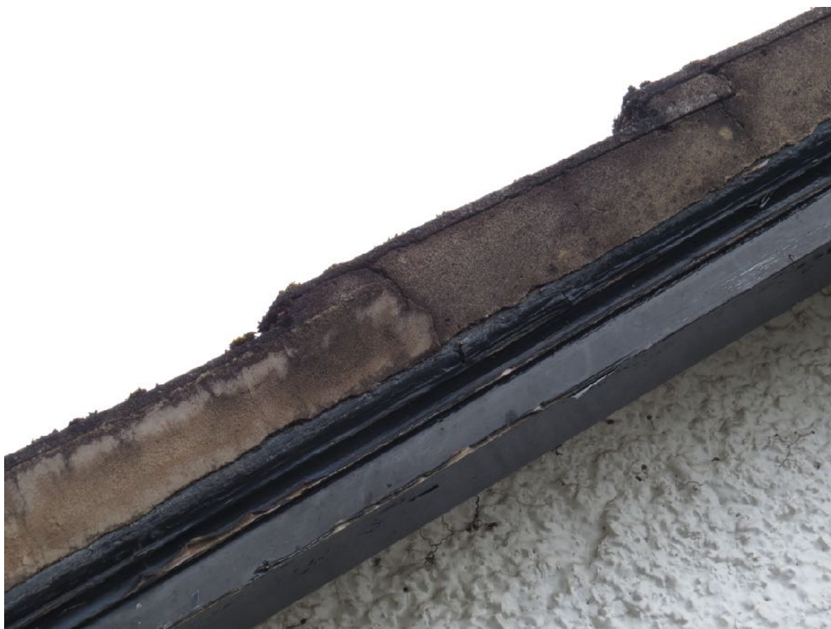
8 – Cement at the verges is in good condition with no suitable gaps.
