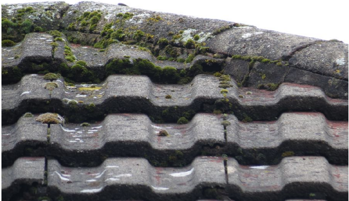
3– Roof and ridge tiles are in good condition with no suitable gaps.
