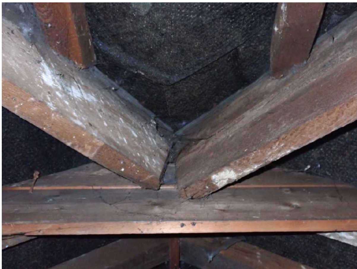
10 – The roof is lined with bitumen felt, joints in timbers are filled with dusty cobwebs.
