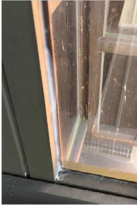
Photograph No. 42 – Clear silicone sealant applied (Level 10 – West elevation – Pall Mall Court)
