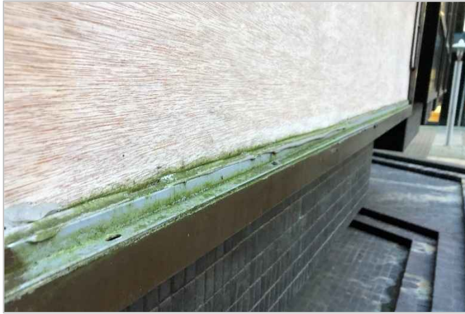
Photograph No. 26 – Timber board installed behind framework and silicone sealed (Level 1 – North elevation – King Street Block)
