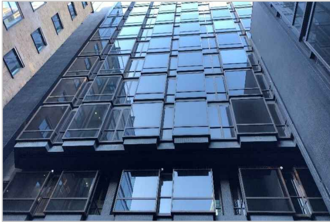
Photograph No. 6 – East elevation – Pall Mall Court Block – Delivery entrance Brown Street
