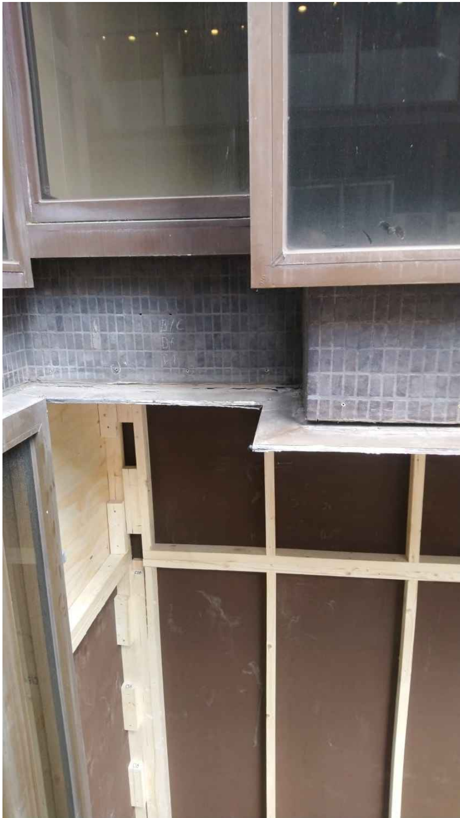
Head pressing cut and left in situ, existing window removed
