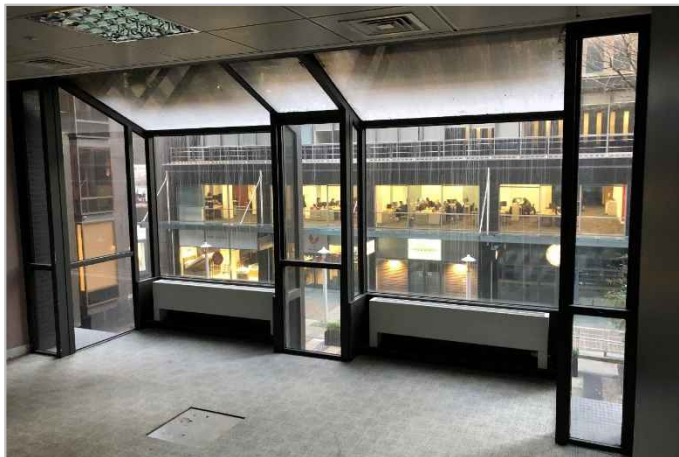
Photograph No. 10 – Two small bay areas on Pall Mall Court Block – Level 1
