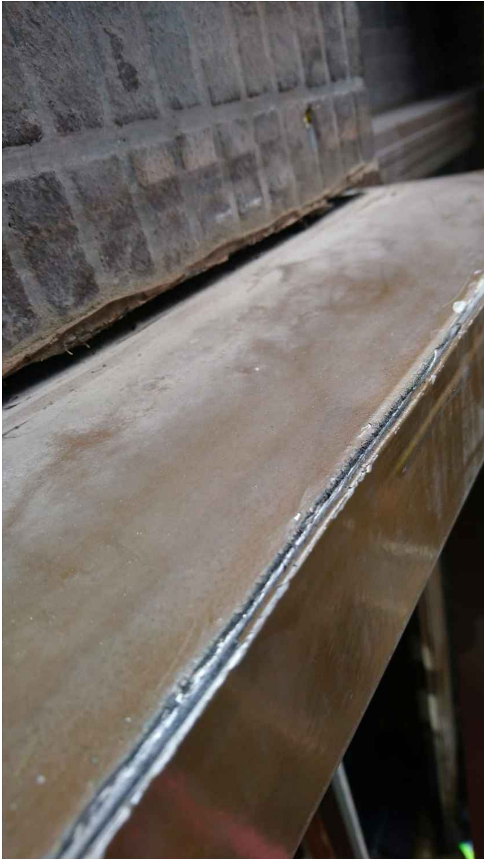
Cut in existing pressing at head of window.
