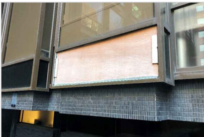
Photograph No. 28 – Timber spandrel panel (Level 1 – North elevation – King Street Block)
