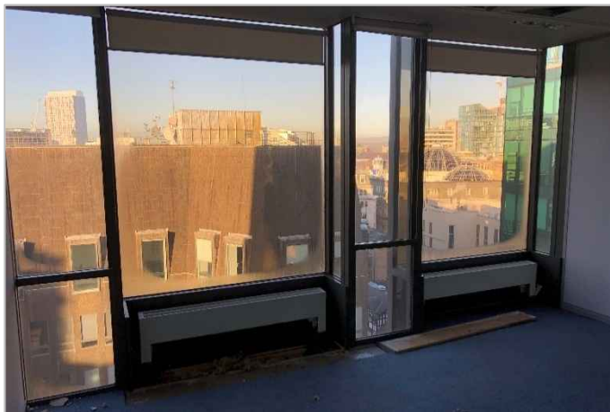
Photograph No. 8 – Continuous bays along elevation with removable partitions – Level 4
