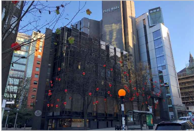
Photograph No. 1 – South elevation – King Street Block – King Street
