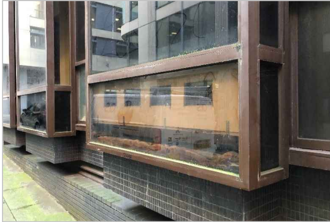
Photograph No. 9 – Aluminium shopfront system installed to all glazing areas
