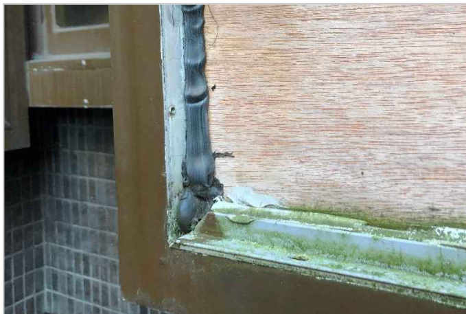
Photograph No. 27 – Timber panel installed, and silicone sealed around the jamb edges (Level 1 – North elevation – King Street Block)
