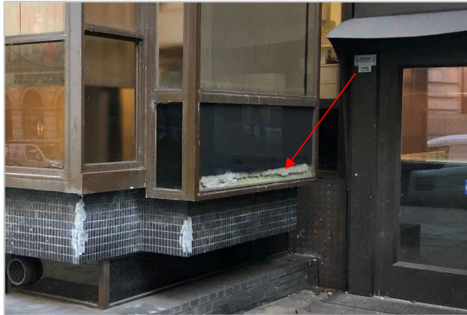
Photograph No. 20 – Spandrel panel on the ground floor (Ground floor – South elevation – King Street)
