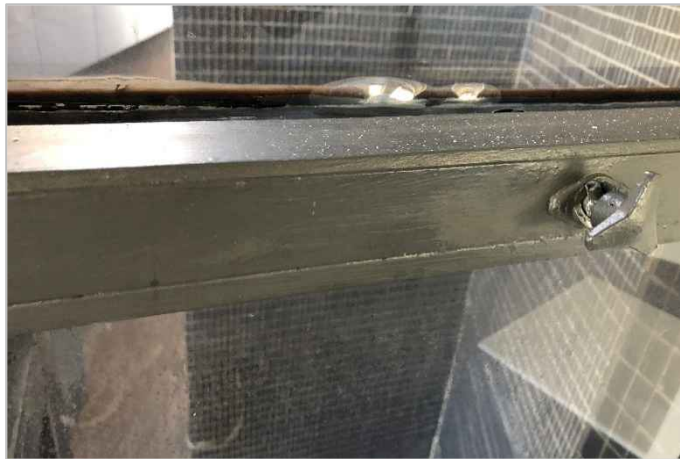
Photograph No. 13 – Film application bubble at window edge
