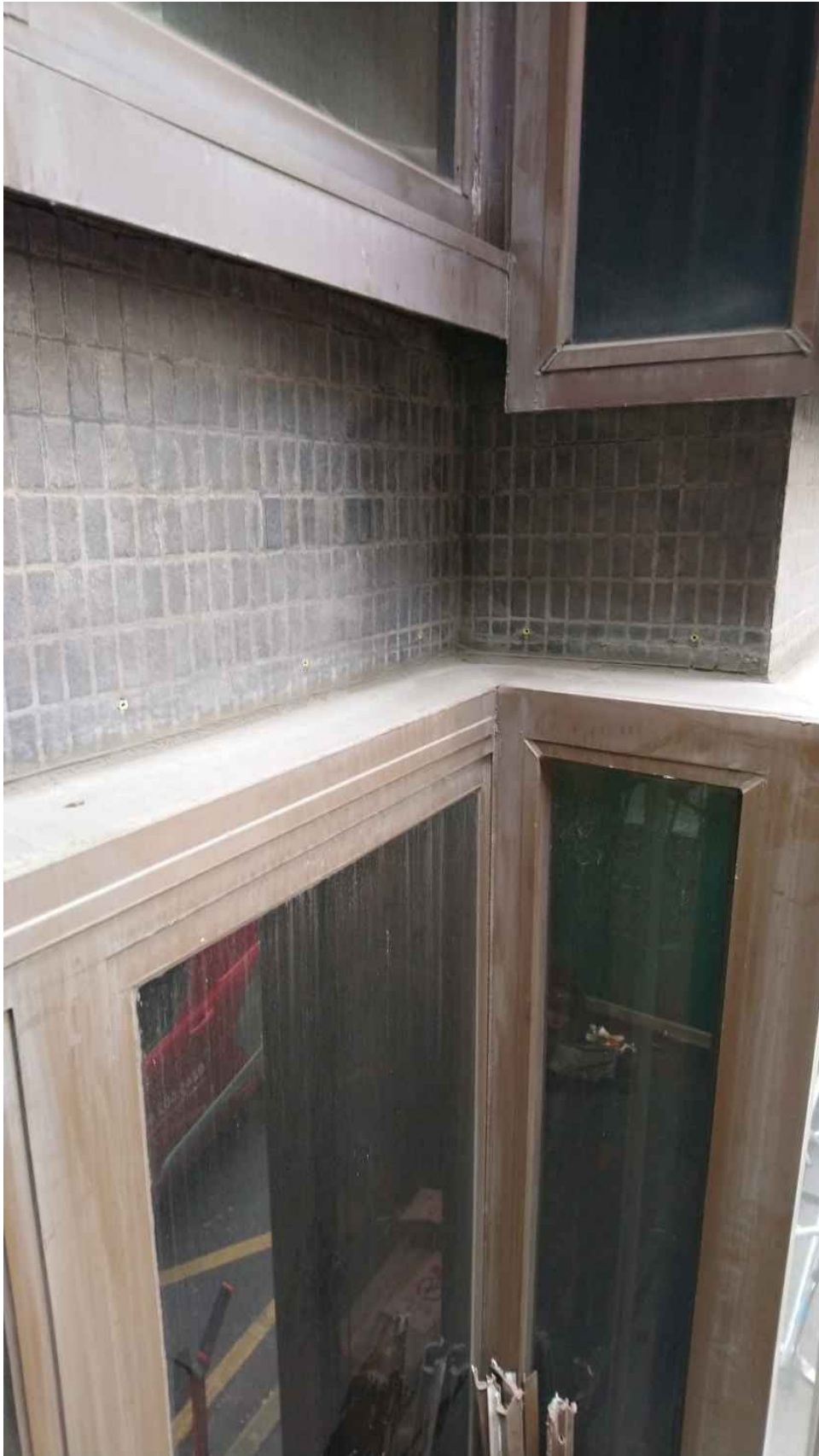
Pressing above window as existing
