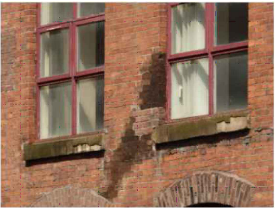
2. Water staining on cornice. Investigate cause and clean. Repoint brickwork with mortar to match existing if necessary.
