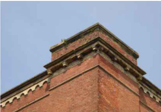
3. High level vegetation to be removed. Brickwork to be cleaned. Repoint brickwork with mortar to match existing if necessary.
