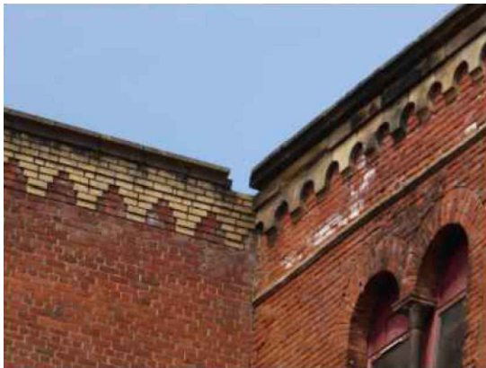
1. Missing section of stone cornice. Replacement stone installed by previous contractor.
