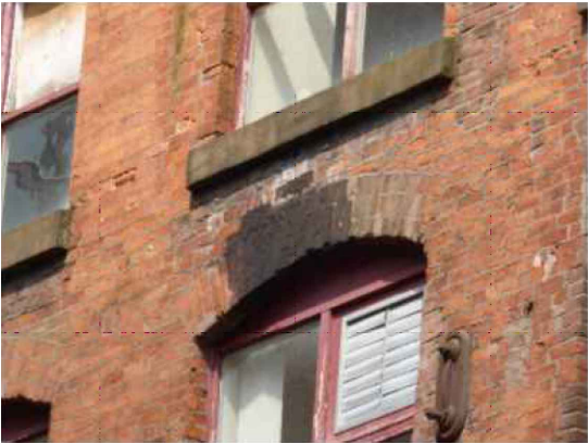
5. Water staining on brickwork. Investigate cause and clean brickwork. Repoint brickwork with mortar to match existing if necessary.
