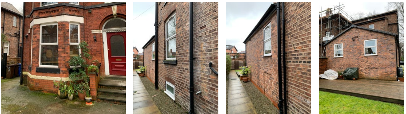
Photographs of Exterior of the Basement
