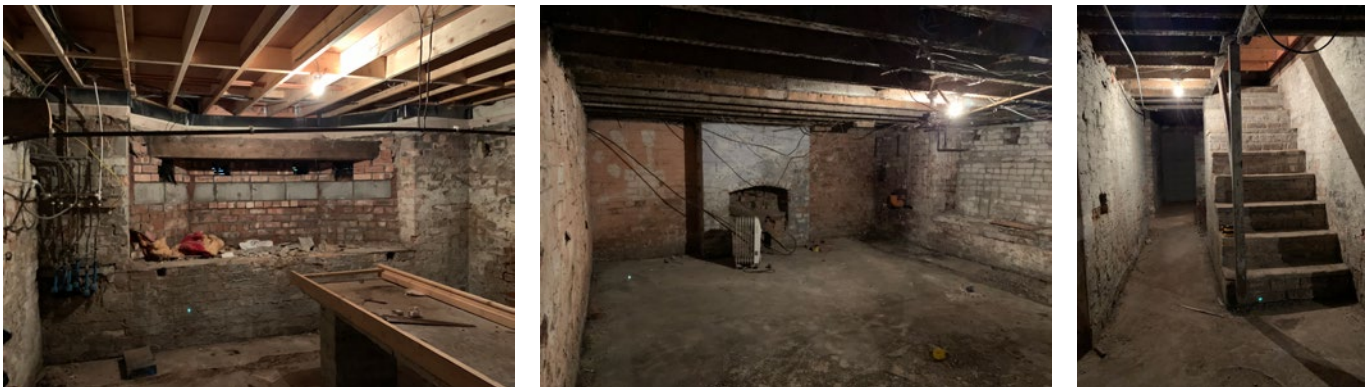
Photographs of Existing Basement (including bricked up bay window)
