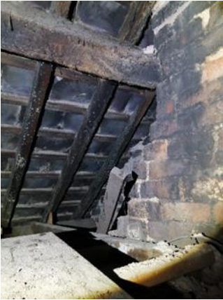
Photograph 14: Partition wall in loft
