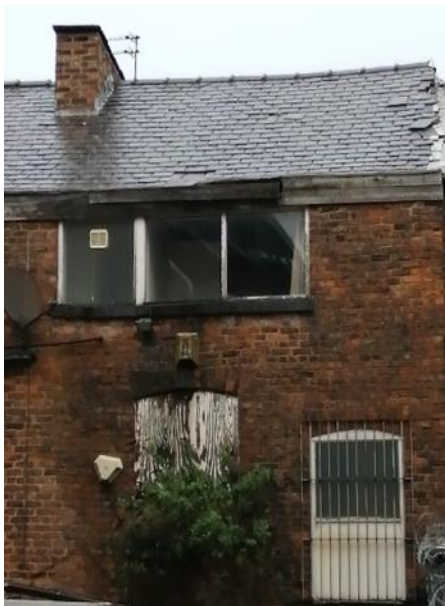
Photograph 3: Southern aspect overview
