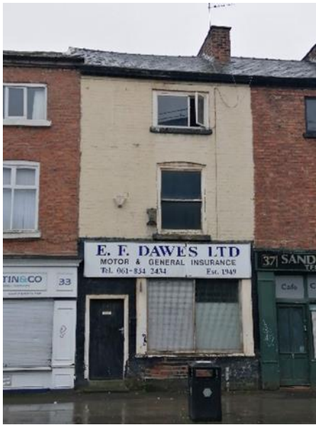
Photograph 1: Northern aspect of B1
