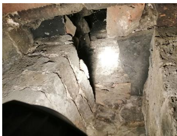
Photograph 11: Connectivity through crevices to other floors
