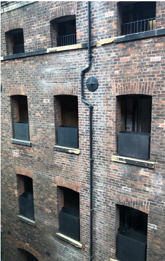
external view of little david street elevation from minshull house
