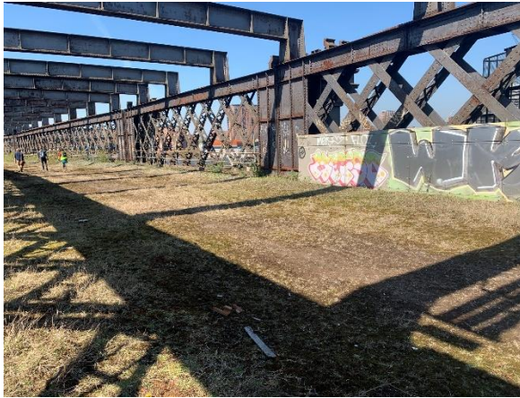
Photograph 1 – Castlefield Viaduct looking west.
