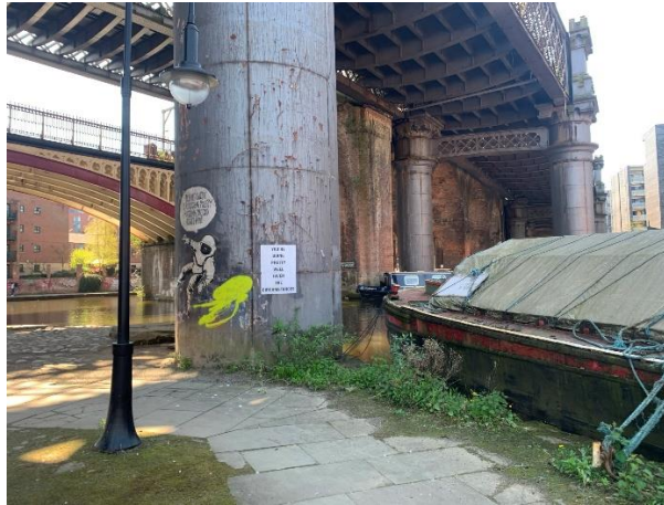
Photograph 2 – Castlefield Viaduct going over the Bridgewater canal.
