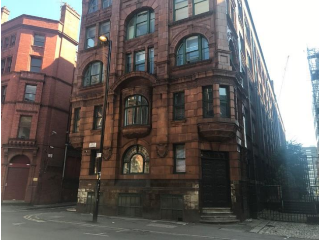
The Langley Building from Dale Street
