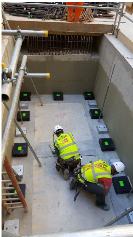
Figure 3 – Mason bearings being placed in one of the core pits. The green labels certifying passing of independent 150% load tests can clearly be seen. We do this for every bearing we make to ensure no risk of failure on site.
