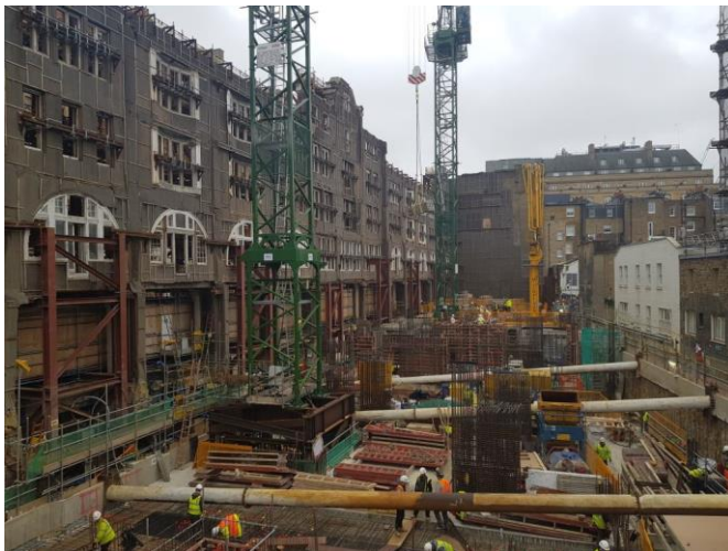
Figure 2 – The cleared site behind the façade
