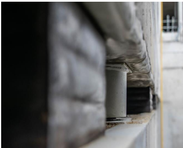
Figure 6: Close up of bearing and lateral restraints
