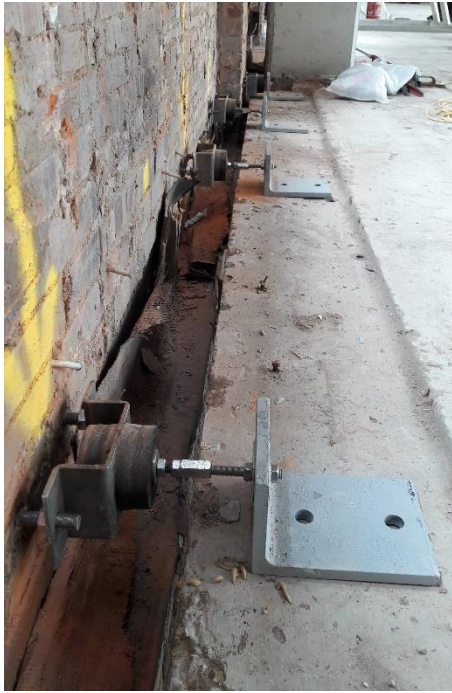
Figure 7: Mason façade ties being installed
