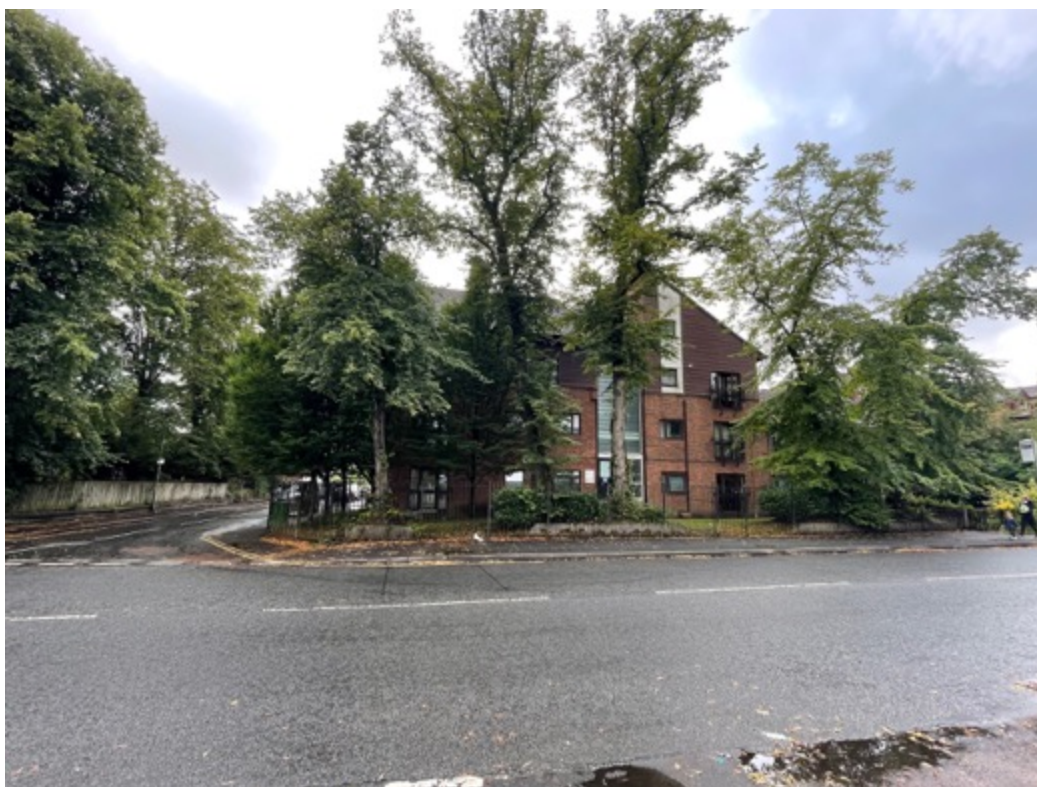
Figure 11- property on the corner of Crumpsall Lane and Polygon Road- directly opposite the application site
