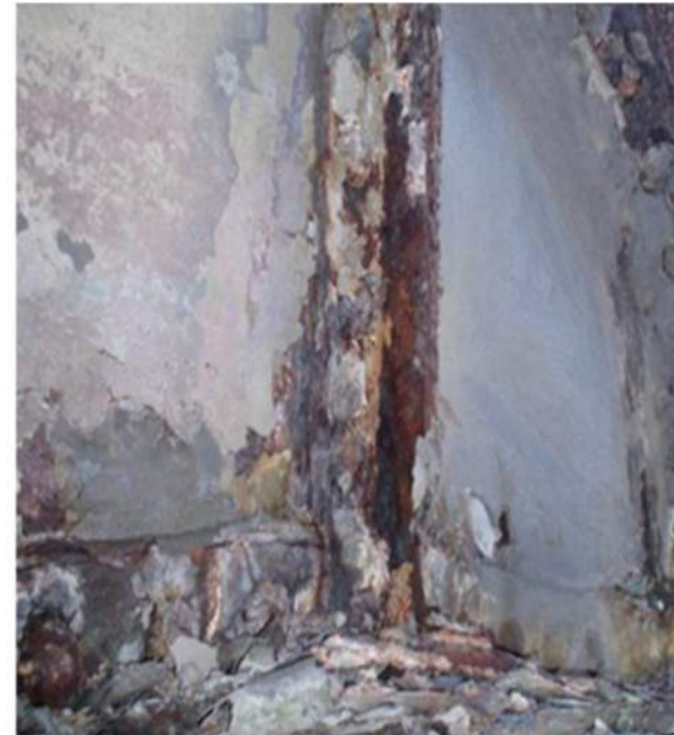
Close up of Stiffener
