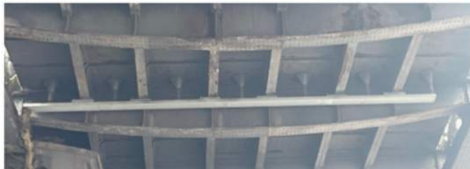
Figure 8 - Example of new drainage channel
