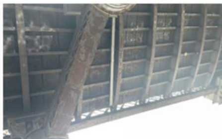
Figure 3 - General condition of the viaduct soffit
