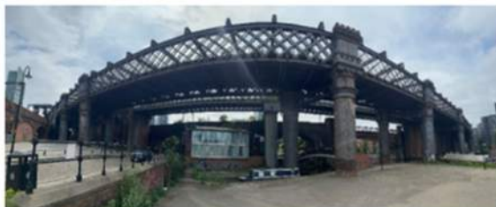
Figure 1 - Overview of viaduct
