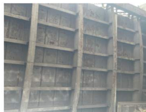
Figure 5 - Typical condition of the deck plate
