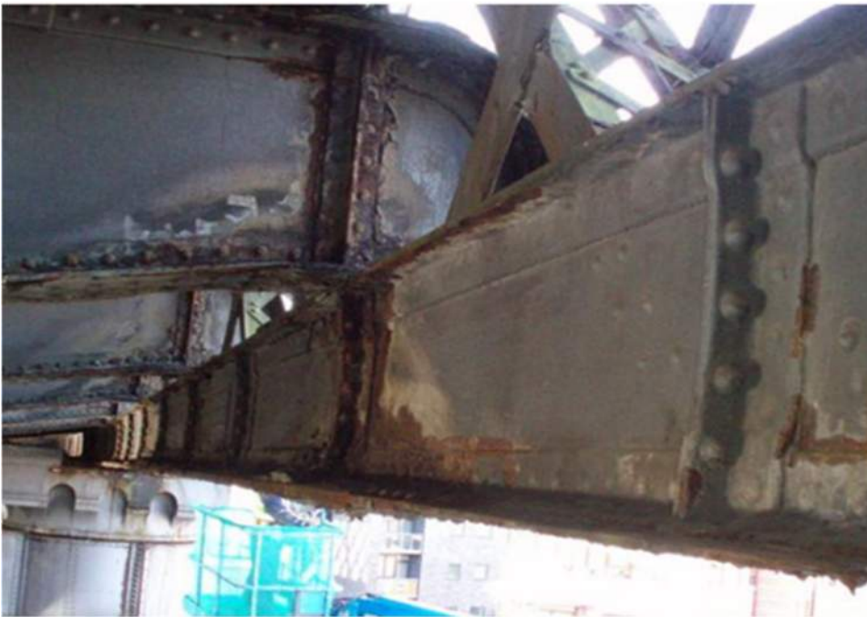
Typical Transvers Girder End Stiffener
