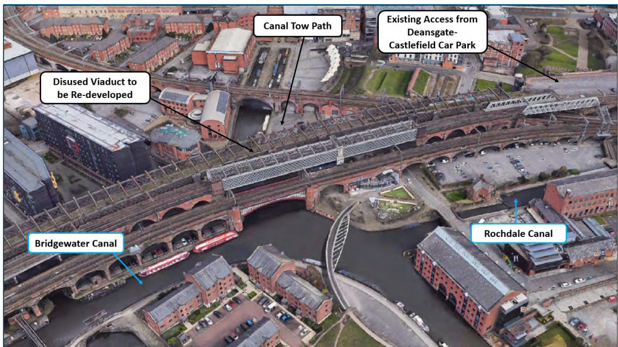
Figure 2-2: Satellite Imagery of Castlefield Viaduct (Source: Twelve Architects Masterplanners)
