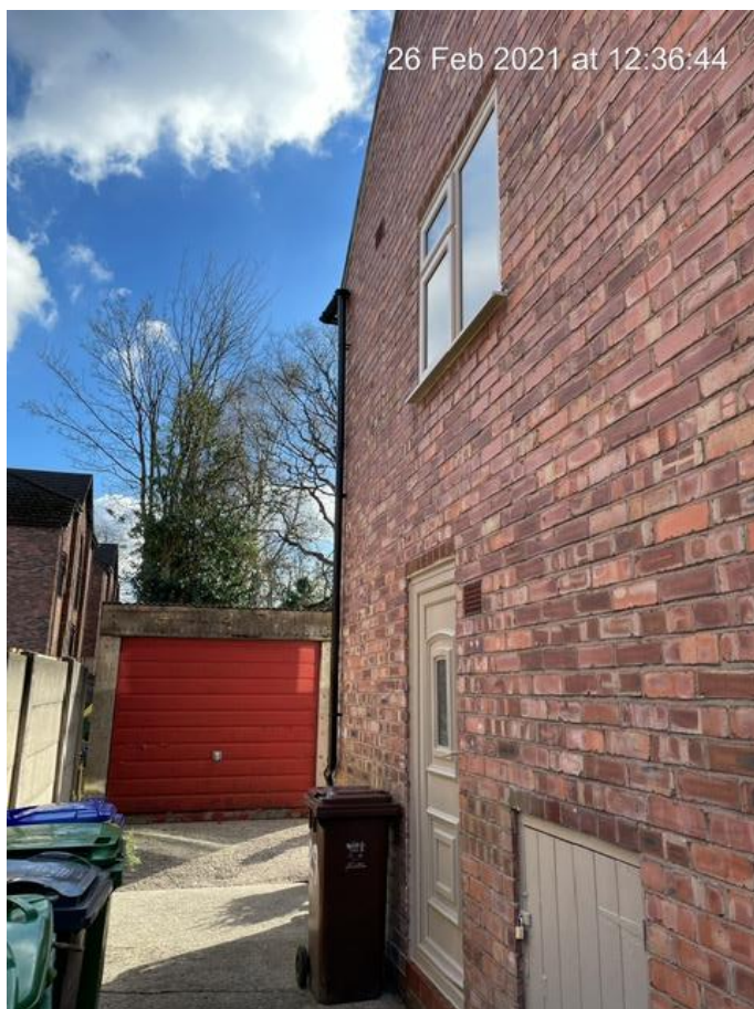
Figure 14 View down side to garage where proposed car port will be erected.
