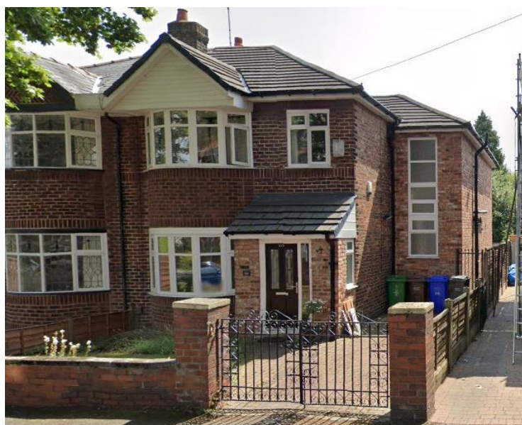
2-storey side extension at No.115 Kingsbrook Road
