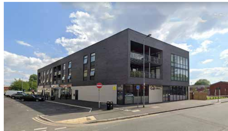
S4B building located opposite the site on Brunswick Street
