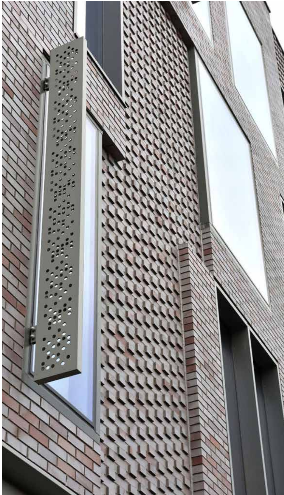
Schuster Annexe building on Upper Brook Street
