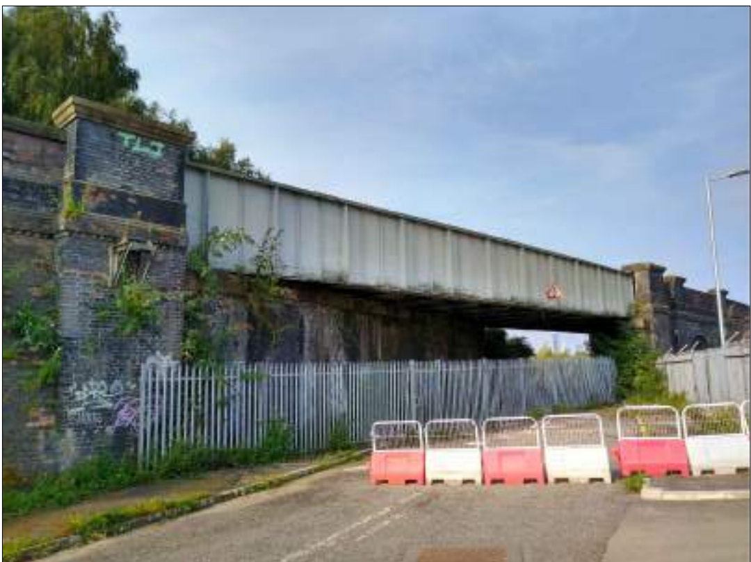
NORTH ELEVATION (PHOTO AS TAKEN IN 2020)
