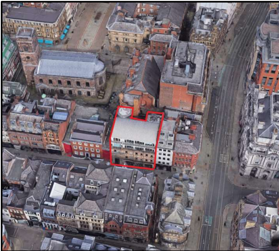
Figure 1: Aerial view of building
