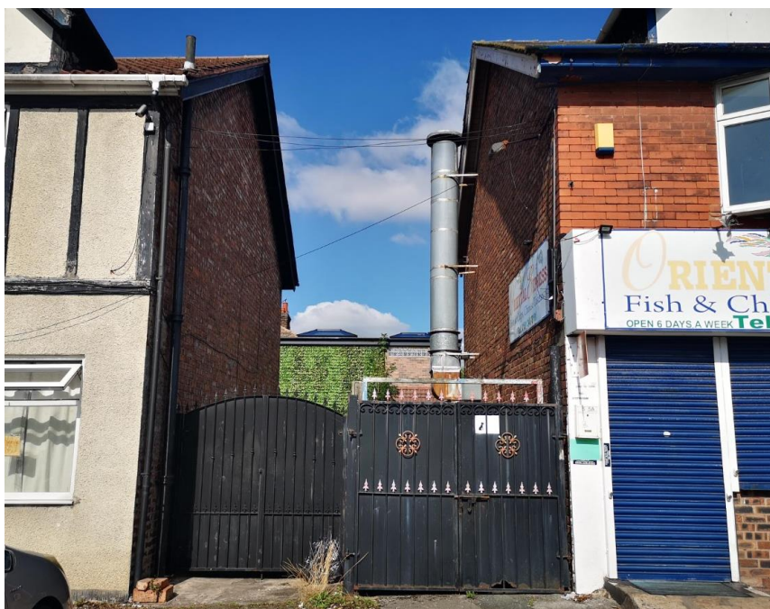
View between properties on Meldon Road towards the current flat roofed two storey extension
