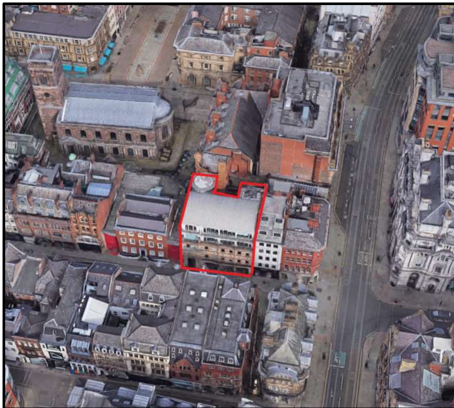
Figure 1: Aerial view of building
