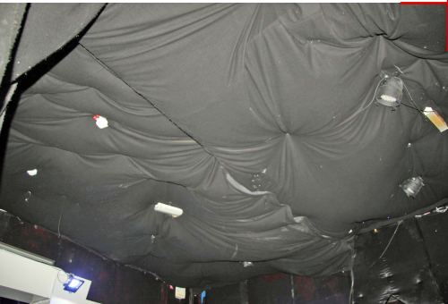
PHOTOGRAPH OF CLUB AREA ADJACENT TO PERFORMING STAGE 1/022 SHOWING FABRIC PINNED TO EXISTING CEILING/SOFFT.
