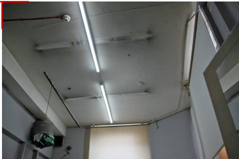
PHOTOGRAPH OF RETROFIT PLASTERBOARD CEILING TO NIGHTCLUB OFFICE AREA. MAJORITY OF FITTINGS ARE SURFACE MOUNTED. ORIGINAL TIMBER BEAMS ARE BOXED IN WITH PLASTERBOARD AND SKIM.
