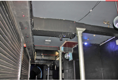
PHOTOGRAPH OF CLUB AREA ADJACENT TO 1/021 BAR SHOWING RETROFIT PLASTERBOARD CEILING AND BOXING OUT OF TIMBER BEAMS. ALL PAINTED BLACK FOR NIGHTCLUB USE. LIGHTS, ALARMS, INDICATORS PREDOMINANTLY SURFACE MOUNTED.
