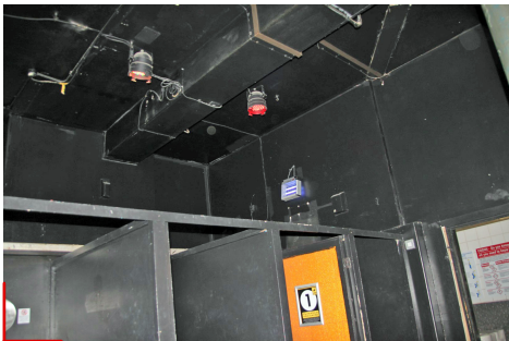
PHOTOGRAPH OF FEMALE WCs 1/011 SHOWING RETROFIT PLASTERBOARD CEILING AND BOXING OUT OF TIMBER BEAMS. ALL PAINTED BLACK FOR NIGHTCLUB USE. LIGHTS, ALARMS, INDICATORS PREDOMINANTLY SURFACE MOUNTED.
