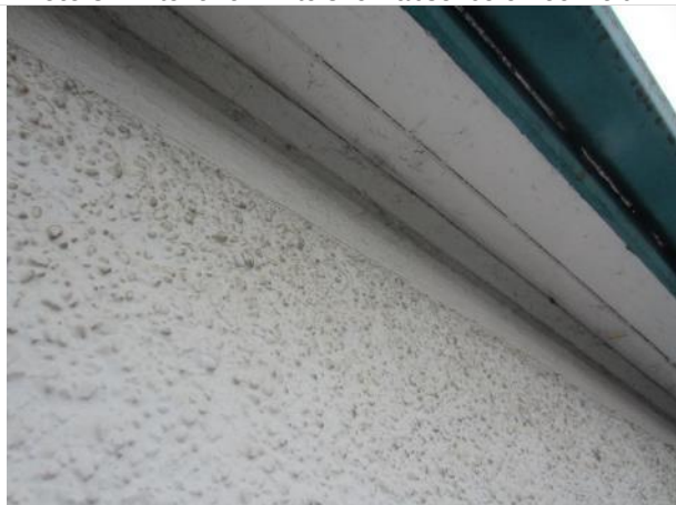
Photo 33: Sealed soffits at B8
