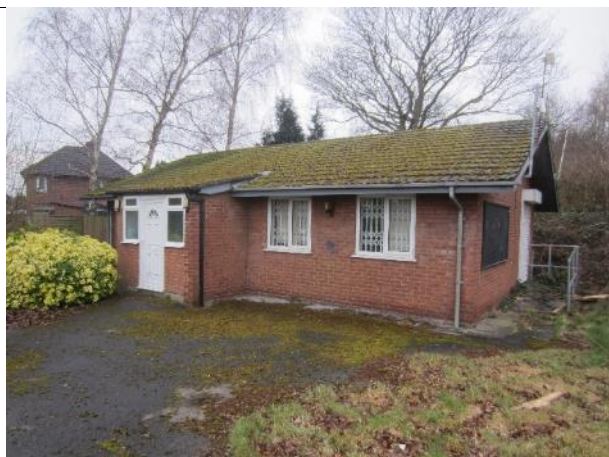
Photo 19: Southern elevation of B4
