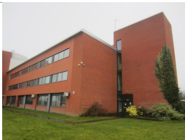
Photo 14: Southern and eastern elevations of B1
