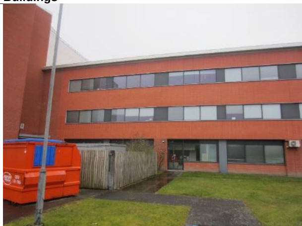
Photo 13: Southern elevation of B1
