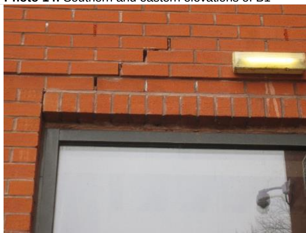
Photo 16: Gaps in brick work at southern elevation of B1; not a potential roost feature
