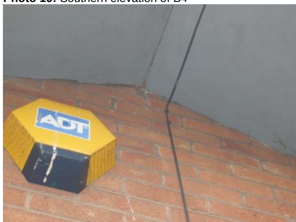
Photo 21: Sealed soffits at gable apex of B4
