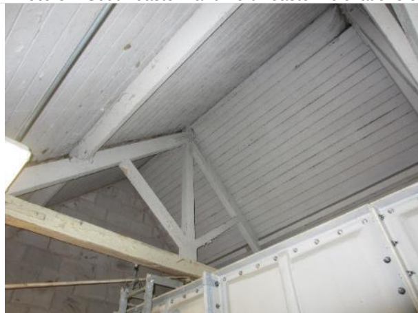
Photo 34: Interior of part of B8 showing timber sarking beneath roof tiles.
