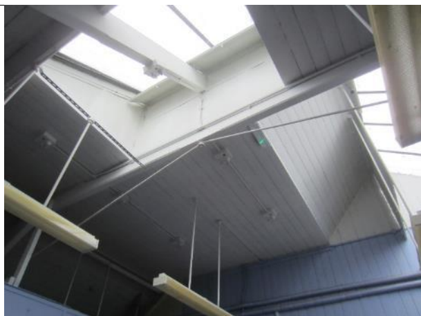
Photo 31: Interior of B7 to show absence of roof void
