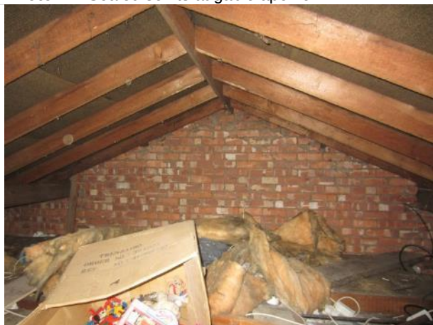
Photo 23: Roof void at B4 (facing east)
