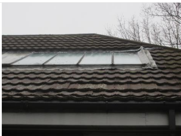
Photo 29: Skylights and flashing at B7
