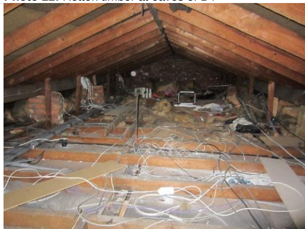
Photo 24: Roof void at B4 (facing west)
