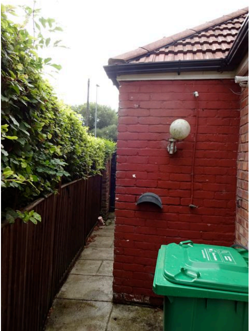
1.12 View of side boundary fence/hedge to 346 Mauldeth Rd West
