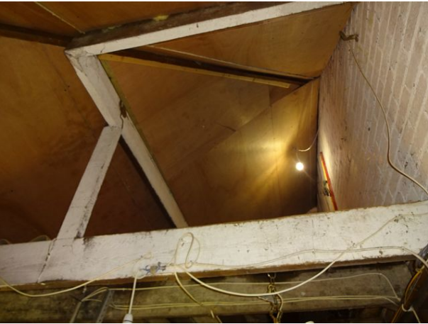
1.11 Internal view of existing garage roof
