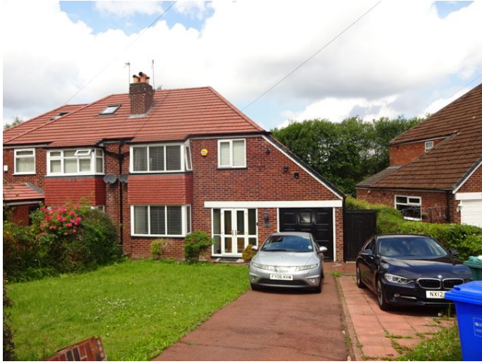
1.1 Front elevation & front garden/driveway facing onto Mauldeth Road West
