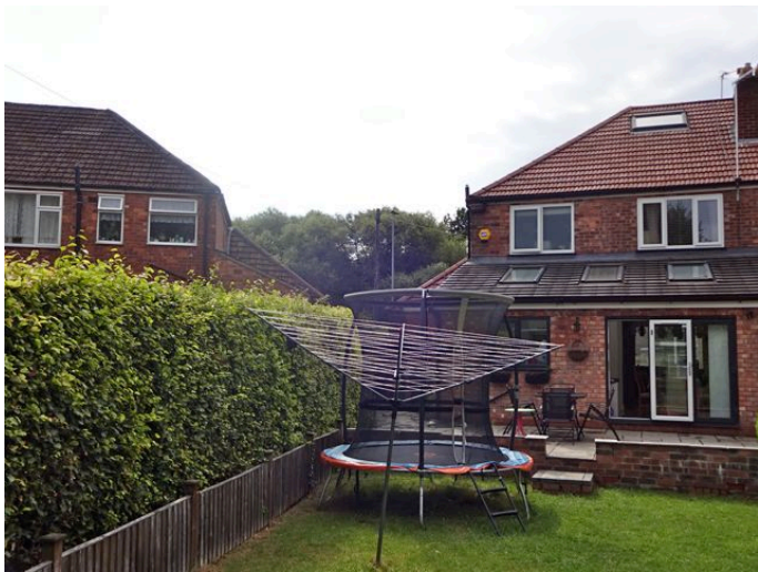
1.3 View of rear elevation with single storey kitchen/dining area facing onto rear garden
