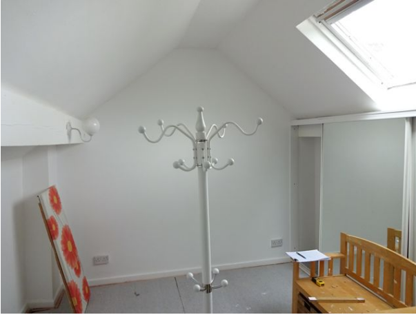
1.10 Internal view of existing loft storage area
