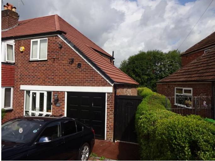
1.2 View of side garage with boundary hedge and 346 Mauldeth Rd West on the right
