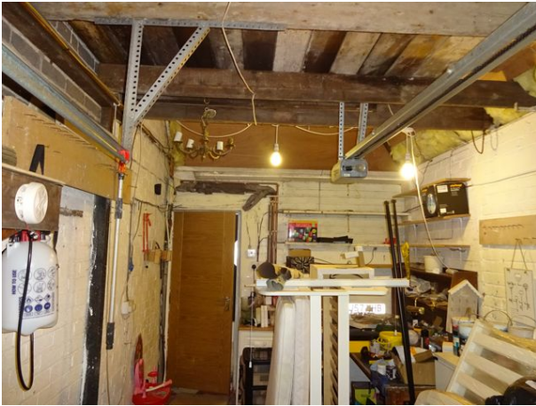
1.8 Internal view of existing garage area
