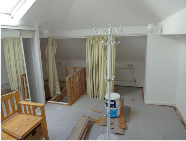
1.7 Internal view of existing loft storage area
