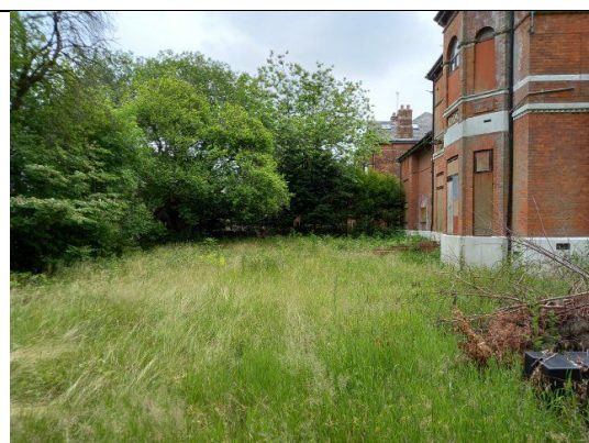
Photograph 4: Northern area of the site, facing east.
