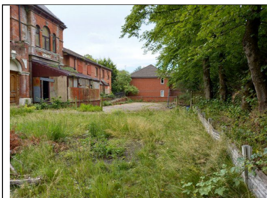
Photograph 3: Western area of the site, facing south.
