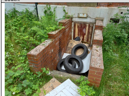
Photograph 5: Entrance to the basement at the northern side of the building.
