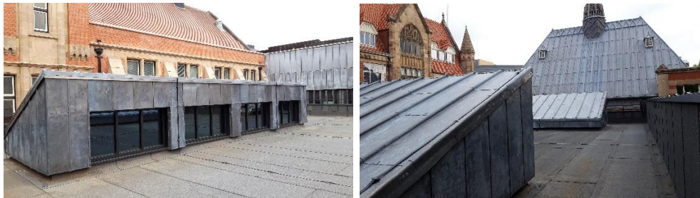
Views of the northlights showing lead cladding and vertical glazing facing north-east.
