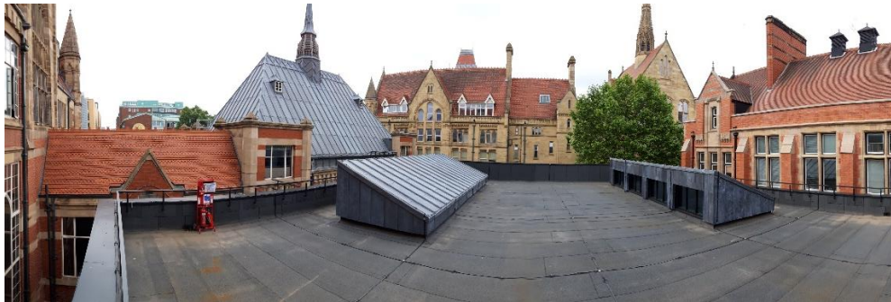
Panoramic view of the newly completed extension roof with the two northlights. Surrounding buildings include (from left) 1927 Museum Building, 1913 Haworth extension, 1911 Haworth Building, 1888 Waterhouse Building and 1901 Rutherford Building
