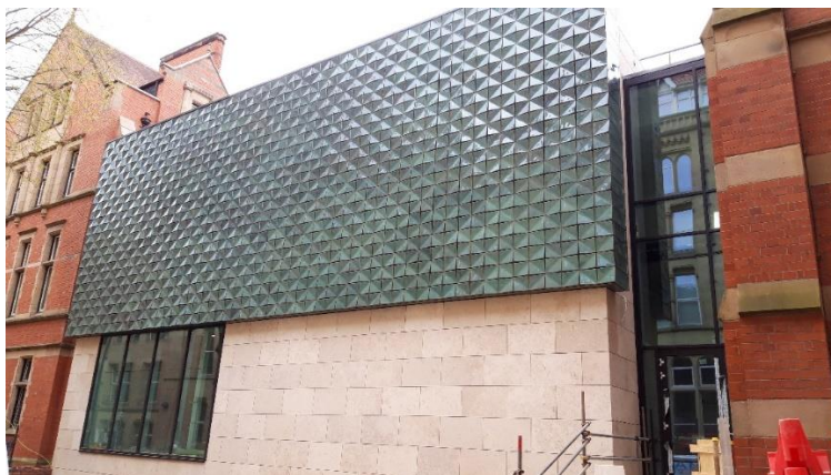
Newly completed Manchester Museum extension. The northlights are located behind the terracotta parapet roof level.
