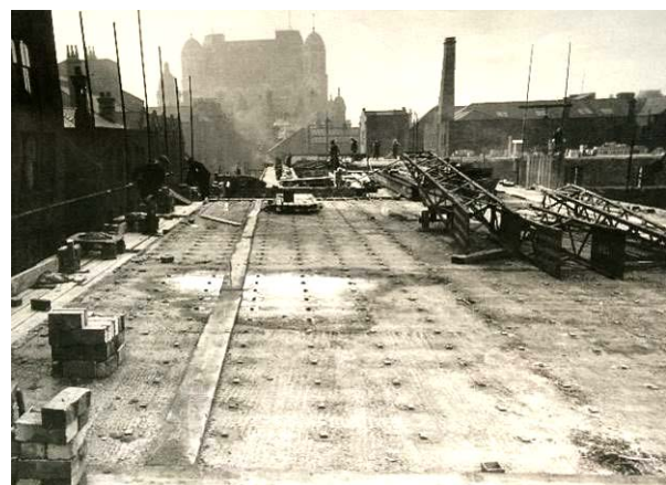
Figure 18: Laying the hollow tile and concrete upper floor c1934.
