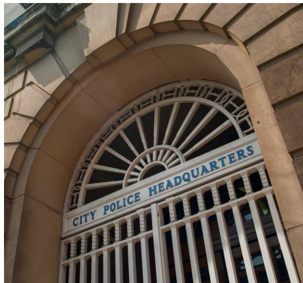
Figure 25: The wrought-iron entrance gates.
