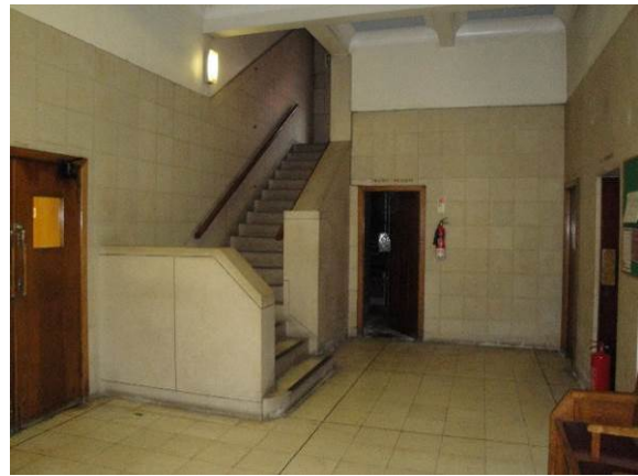
Figure 45: The basement floor hall showing the terrazzo stairs and flooring.
