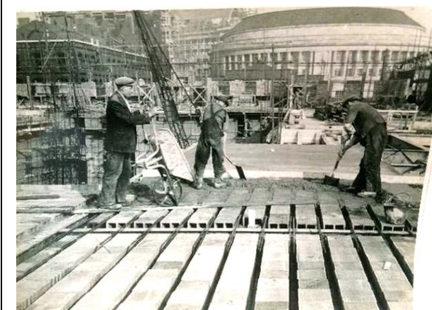
Figure 17: Laying the hollow tile and concrete ground floor c1934.
