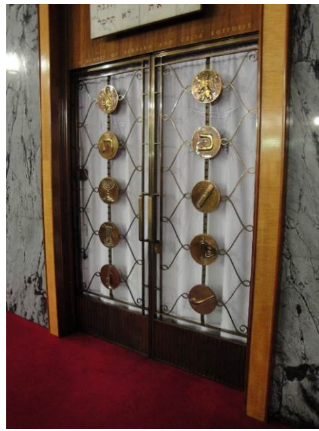
Figure 47: The Ark is situated to the centre of the room and is constructed of a grey/green marble with filigree iron and brass doors.
