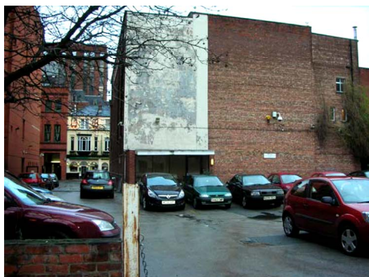
Figure 42: The rear (south) elevation as viewed from Bootle Street.
