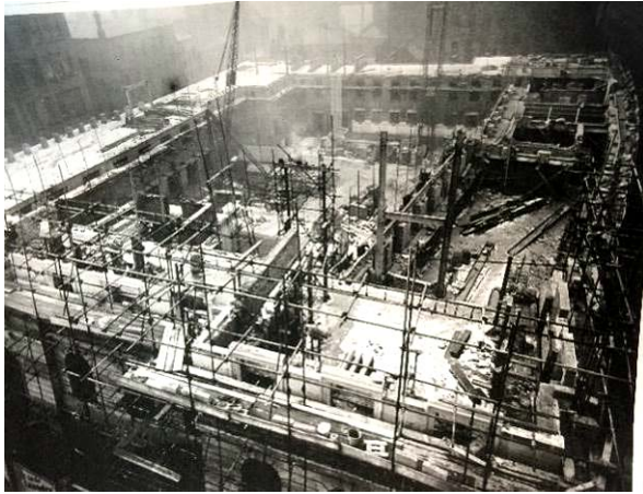
Figure 19: Constructing the upper floors of the building Feb 1936
