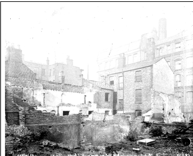
Figure 15: A view looking from South Street across the partially cleared former fire station site in preparation for the laying of the Police Headquarters, 29 th October 1933.
