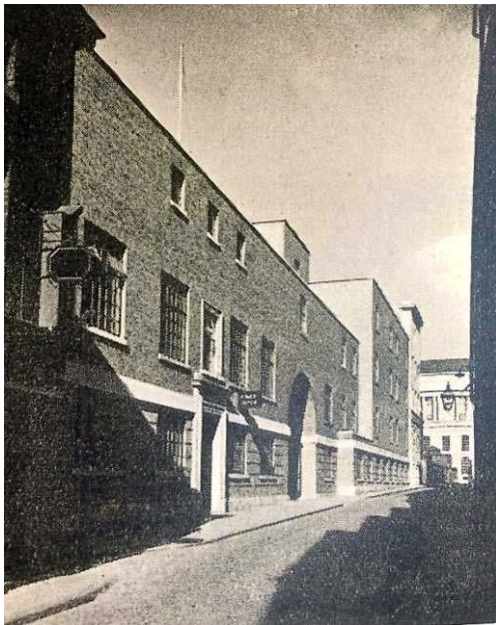
Figure 21: Looking east along Bootle Street towards South Street in 1937, showing the newly completed building to the left.
