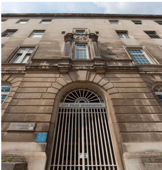
Figure 24: Detail of Southmill Street elevation, 2014
