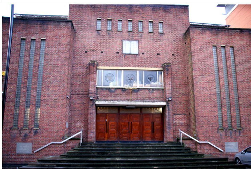
Figure 40: The north elevation as seen from Jacksons Row.
