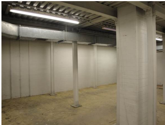
Figure 36: a typical room in the east end of the basement, 2015.
