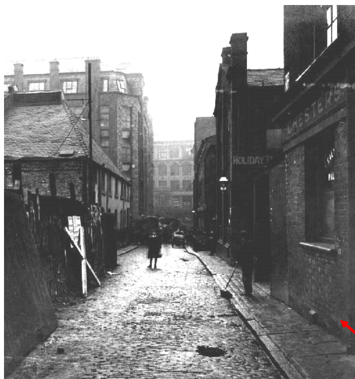
Figure 10: A view looking west along Bootle Street towards Deansgate in the early 20th Century. The corner of the Abercromby can be seen on the extreme right, showing a member of staff sweeping out the attached barrel-run lean-to. Note the early window sills and windows on the ground floor. These have been replaced.
