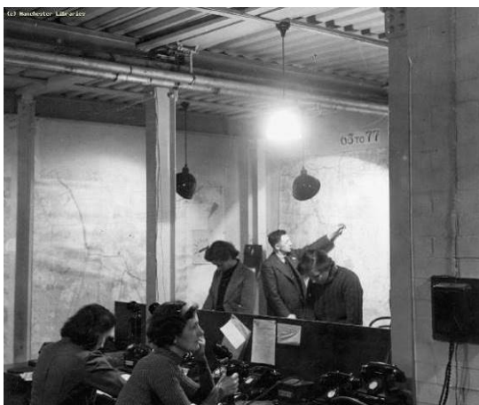
Figure 32: Police switchboard staff seen in the main control room in 1940. Note the strengthened corrugated ceiling.
