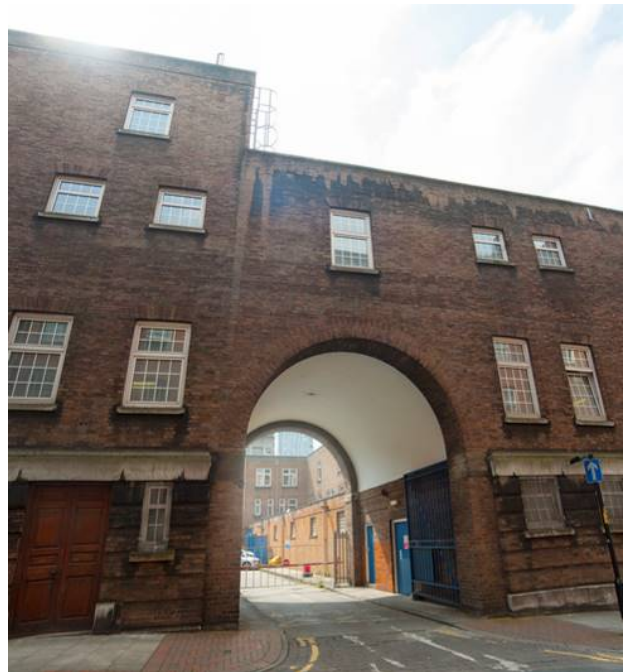
Figure 27: The Jackson's Row arched entrance into the central courtyard. Note the original paneled doors to the left.
