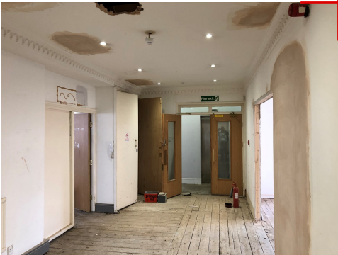
PHOTOGRAPH OF CIRCULATION LOBBIES AND PARTIALLY COMPLETED WC'S SHOWING HOW THE EXISTING FLOOR JOISTS ABOVE HAVE BEEN UNDERDRAWN WITH MODERN PLASTERBOARD AND SKIM FINISH, PAINTED WITH WHITE EMULSION AND THE SUBSEQUENT INSTALLATION OF MODERN SPOT DOWNLIGHTERS. CORNICE TO CIRCULATION LOBBY IS NON-ORIGINAL.
