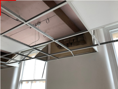
PHOTOGRAPH OF SUSPENDED CEILING WITH CUT-BACK TO ACCOMMODATE WINDOW HEADS AT GREATER HEIGHT
