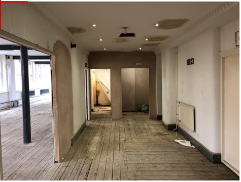
PHOTOGRAPH OF CIRCULATION LOBBIES AND PARTIALLY COMPLETED WC's SHOWING HOW THE EXISTING FLOOR JOISTS ABOVE HAVE BEEN UNDERDRAWN WITH MODERN PLASTERBOARD AND SKIM FINISH, PAINTED WITH WHITE EMULSION AND THE SUBSEQUENT INSTALLATION OF MODERN SPOT DOWNLIGHTERS. THE WALL ON THEIR RIGHT IS THE ORIGINAL SPINE WALL. THE WALL ON THE LEFT IS A MODERN PARTITION.
