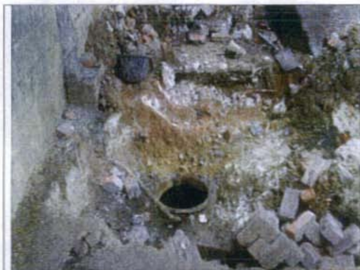
Photograph 1 Top of the tank
