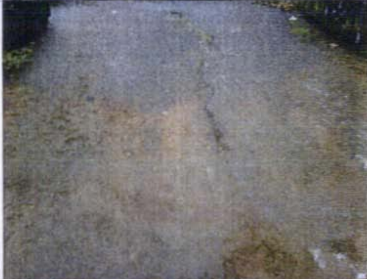
Photograph 8 Intact hardstanding looking east towards WS3
