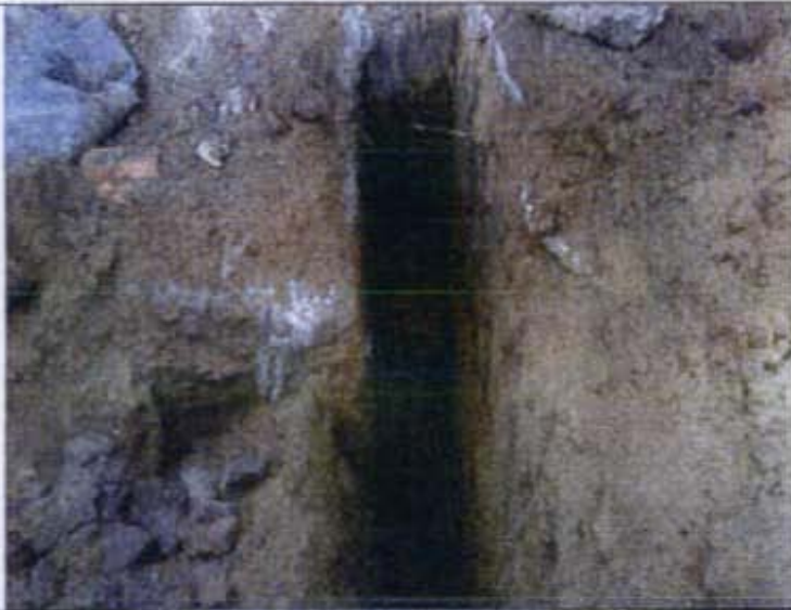
Photograph 7 TP101 Concrete bunding can be seen at the rear face of excavation
