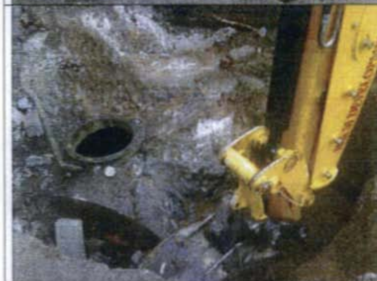
Photograph 2 Excavating around the tank to confirm extent
